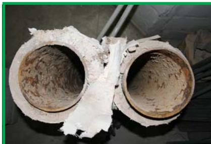
*Contractors installing the new HVAC system throughout the Capitol are replacing worn, corroded pipes such as these.*
