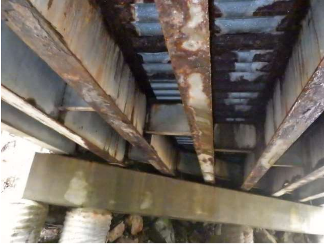
Typical underside of deck
