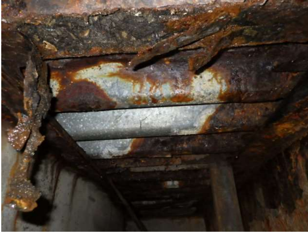
Failed area of decking where next hole is possible
