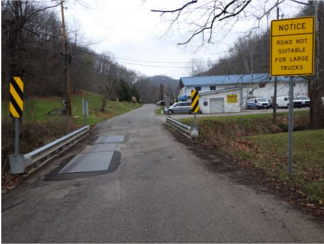
Top of bridge deck with multiple repairs.
