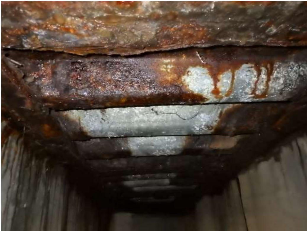
Existing rusting decking
