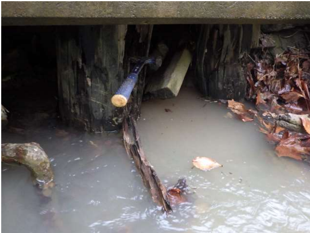
Severe rot, typical of all piles that are exposed
