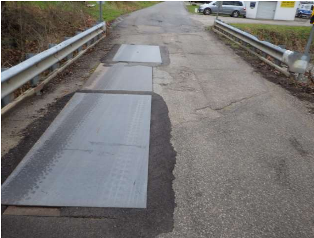
Previous failures covered in plates, which could puncture tires if repair material comes loose around them and are often slick in the winter, posing a risk for accidents.
