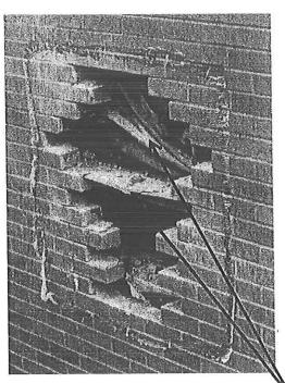
Note that the flashing is torn and forward edge of the flashing is located about 1" back from the face of the wall. This allows any water which had been caught by the flashing above to drain back down into the wall, rather than out across the face. Flashing is also not well secured to the backup.
