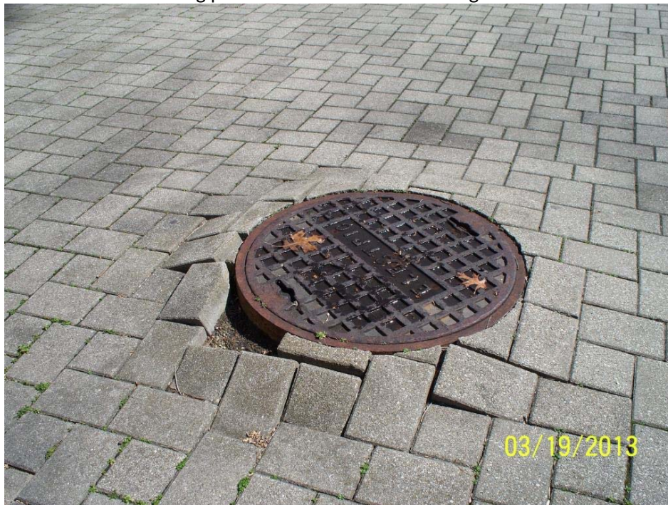
33. Uneven and missing pavers around manhole on stage north of the fountain circle.
