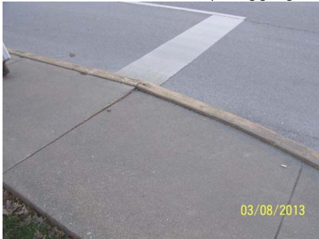
18. Sunken concrete north side of parking garage has created lip at curb.
