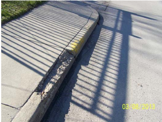
17. Damaged curb near guardshack on Piedmont St.
