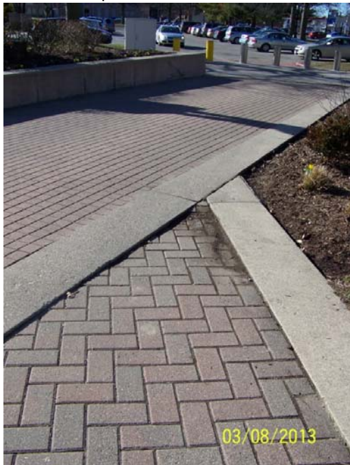
10. Uneven pavers at Coal Miner Memorial.
