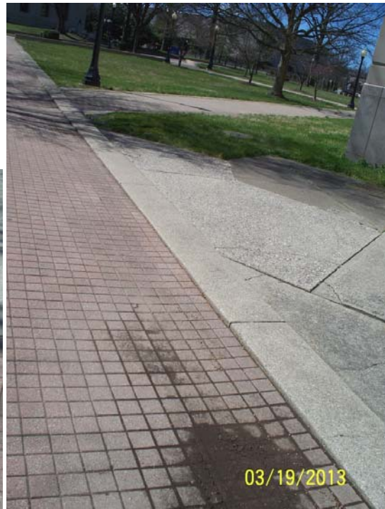
33. Uneven and missing pavers around manhole on stage north of the fountain circle.
