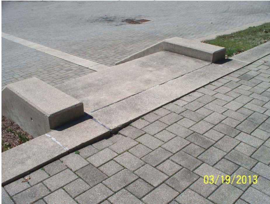
34. Sunken pavers at stairs leading from stage north of the fountain circle.
