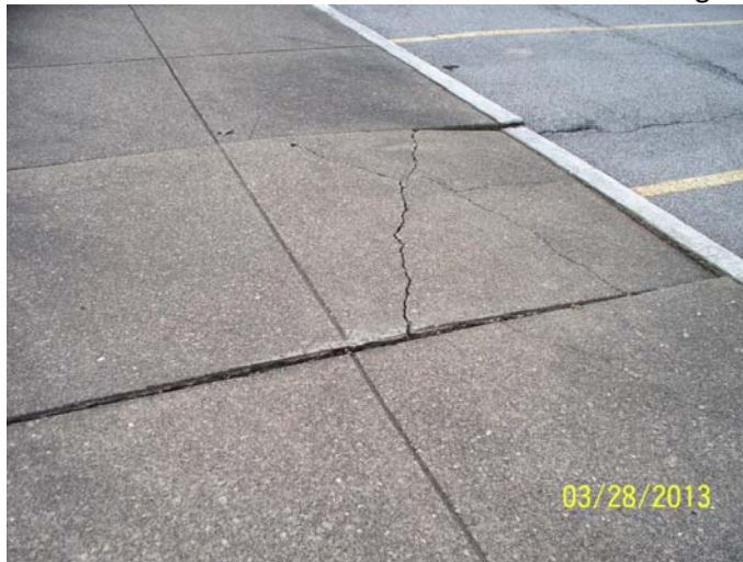
40. Sunken and broken concrete on sidewalk east of guardshack.
