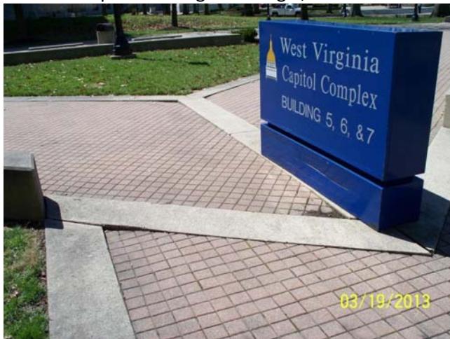
23. Sunken pavers at Sign for Bldg 5, 6 and 7.
