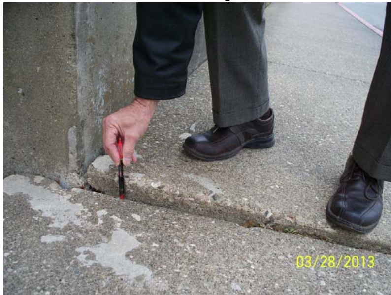
41. Uneven sidewalk north side of Bldg 3.
