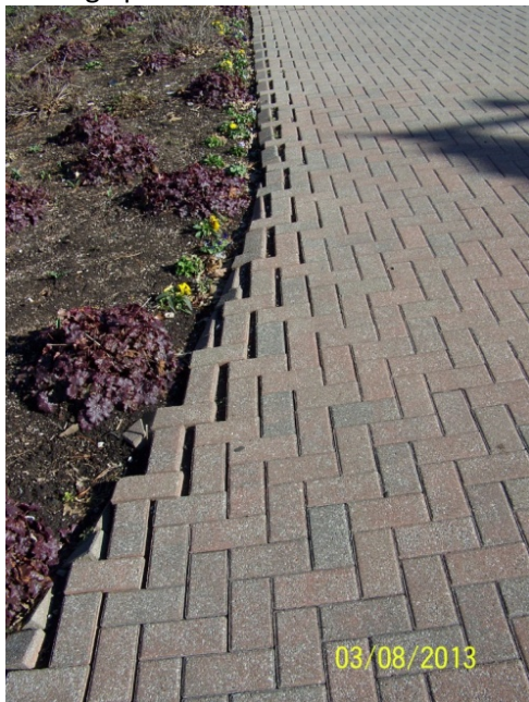
13. Edge pavers at Greenbrier St entrance have fallen over.
