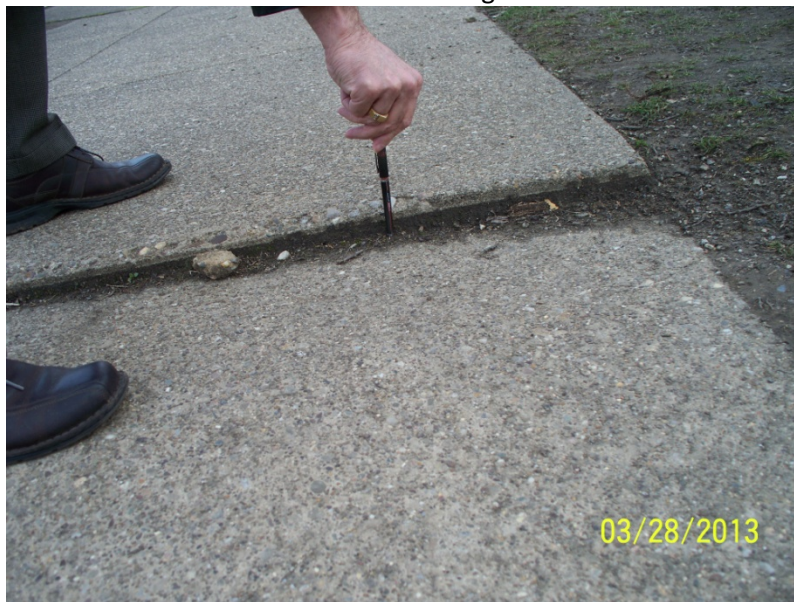
39. Raised concrete on sidewalk east of guardshack.
