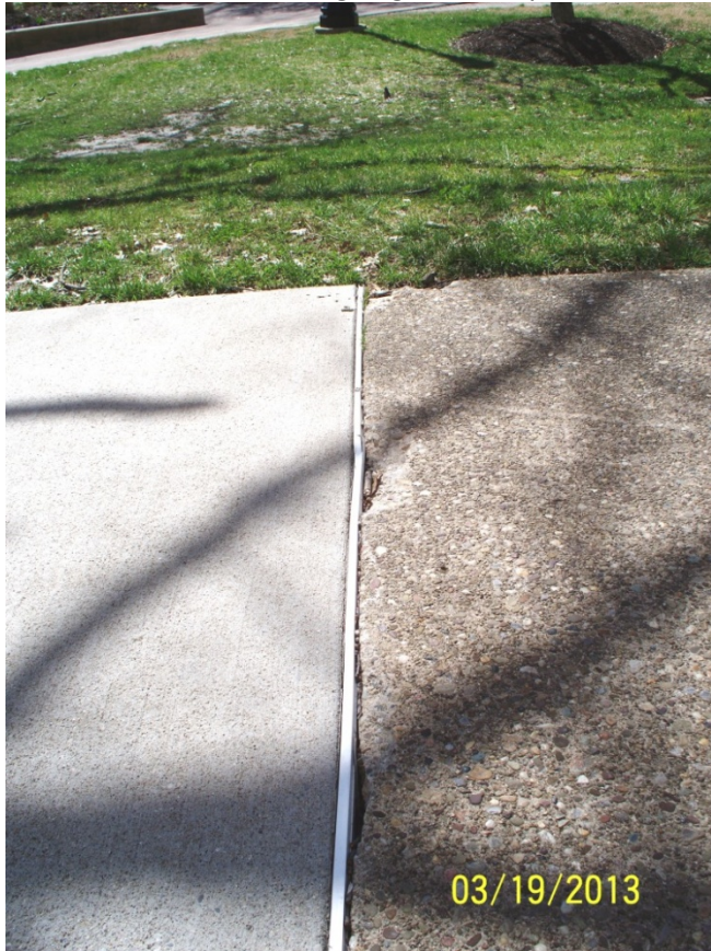
26. Concrete broken along edge walkway south side of Bldg 6.
