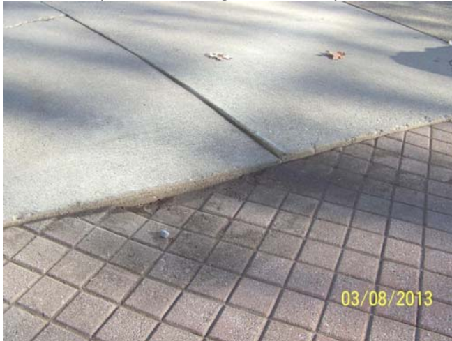
20. Sunken pavers at triangle in walkway entrance from CA Street, southwest corner of Building 6.
