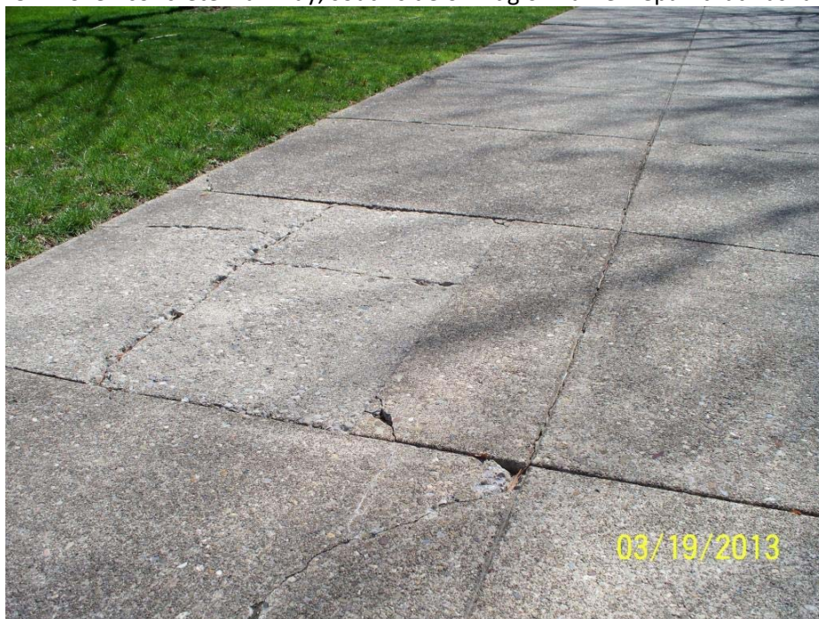
25. Broken concrete walkway, south side of Bldg 6. Earlier repair that has failed.
