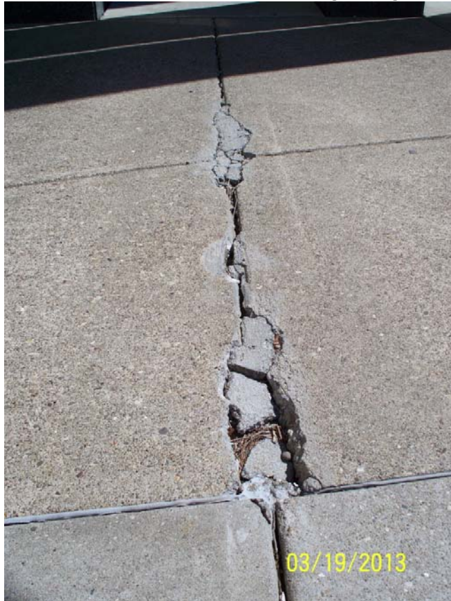
28. Concrete cracked at entrance to Bldg 7, Bldg 5 side. Earlier repair has failed.
