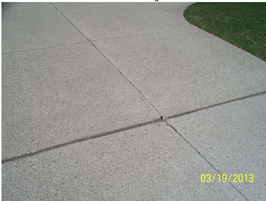
31. Sunken concrete at west entrance to Bldg 5.
