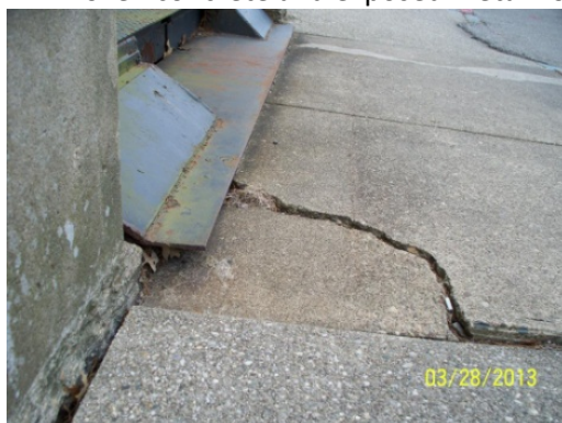
42. Broken concrete and exposed metal north side of Bldg 3.
