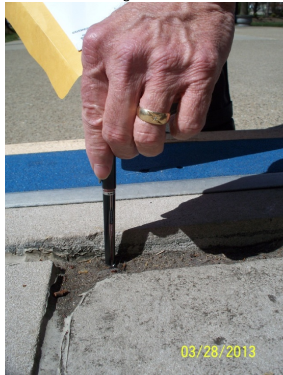
36. Lip at stairs and large gaps in stones at Governor's entrance to Bldg 1.
