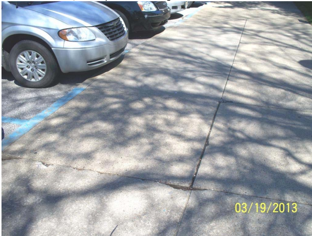
30. Broken concrete, walkway west side of Bldg 5.
