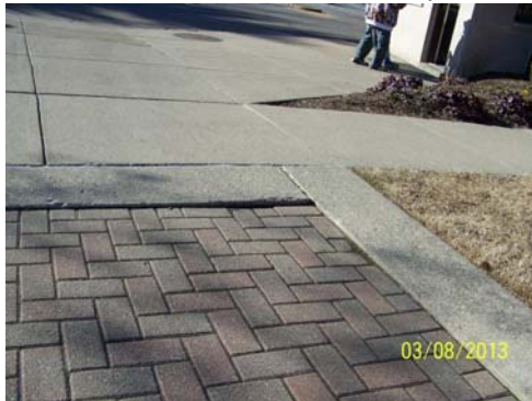
12. Pavers have sunk on walkway at Greenbrier St entrance.
