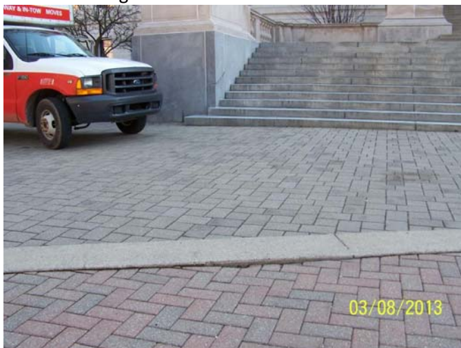
22. Pavers have sunk in relation to concrete on all the walkways surrounding the fountain on the north side of Bldg. 1.
