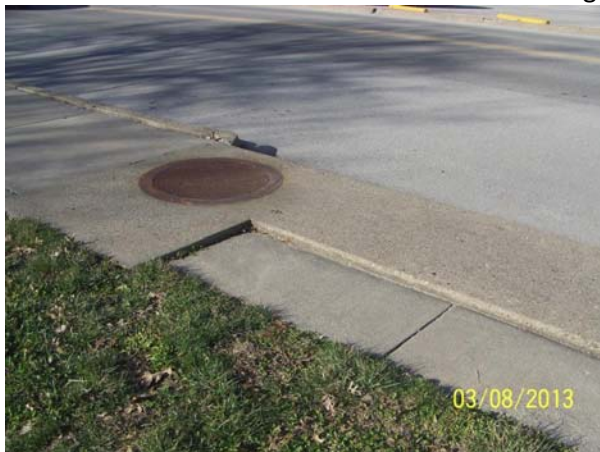
19. Uneven sidewalk at manhole near Piedmont guardshack.
