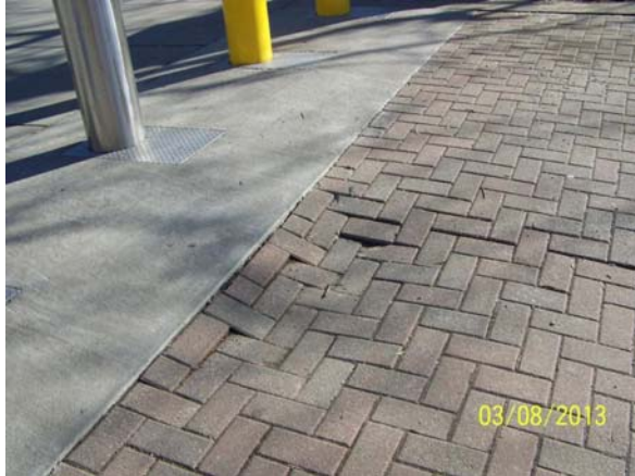
12. Pavers have sunk on walkway at Greenbrier St entrance.
