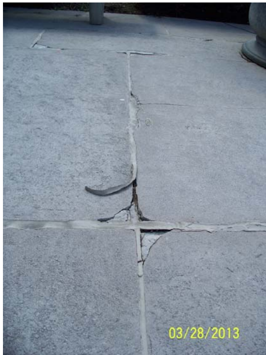
36. Lip at stairs and large gaps in stones at Governor's entrance to Bldg 1.
