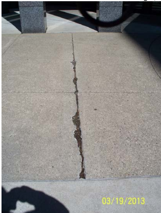
27. Concrete cracked at entrance to Bldg 7, Bldg 6 side.
