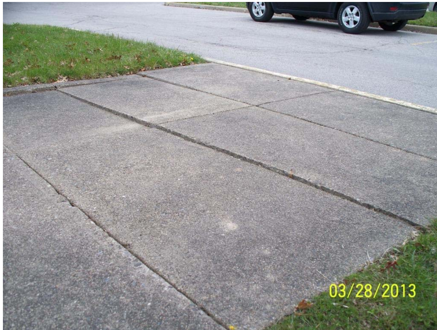
39. Raised concrete on sidewalk east of guardshack.
