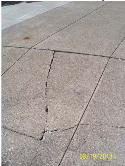
29. Broken, sunken concrete at Bldg 5 south side entrance.
