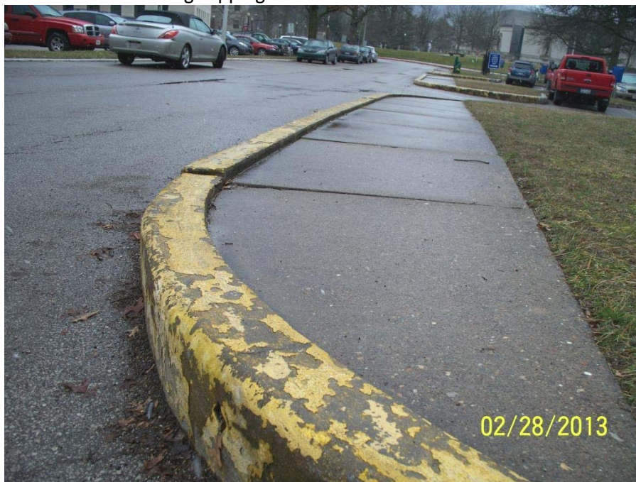
37. Sidewalk sections at the end of parking islands running east to west, on east side of parking garage have sunk creating tripping hazards at curbs.
