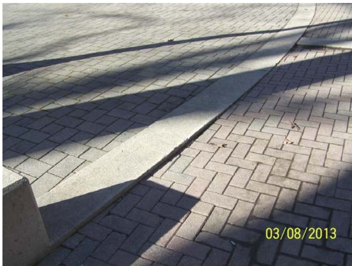
23. Sunken pavers at Sign for Bldg 5, 6 and 7.
