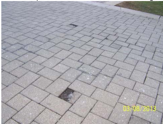
22. Pavers have sunk in relation to concrete on all the walkways surrounding the fountain on the north side of Bldg. 1.
