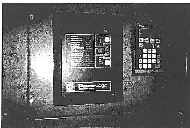
Photo 3D-1 Monitor Indicating THD(I) Reading of 7.9%
