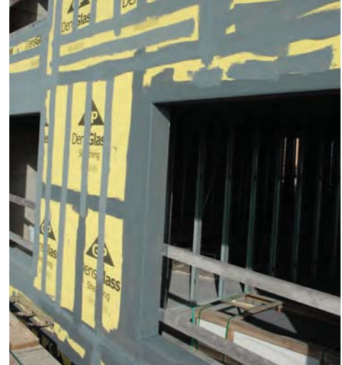
ENERSHIELD and SHEATHING FABRIC combine to create self gauging window flashings custom molded for each window and seamlessly integrated into the air/water-resistive barrier.
