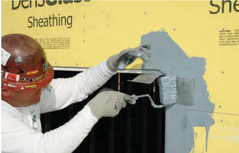
ENERSHIELD and SHEATHING FABRIC combine to create self gauging window flashings custom molded for each window and seamlessly integrated into the air/water-resistive barrier.
