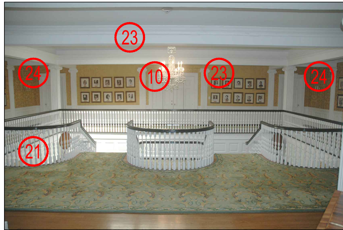
W - 2nd Floor Reception Room North Wall
