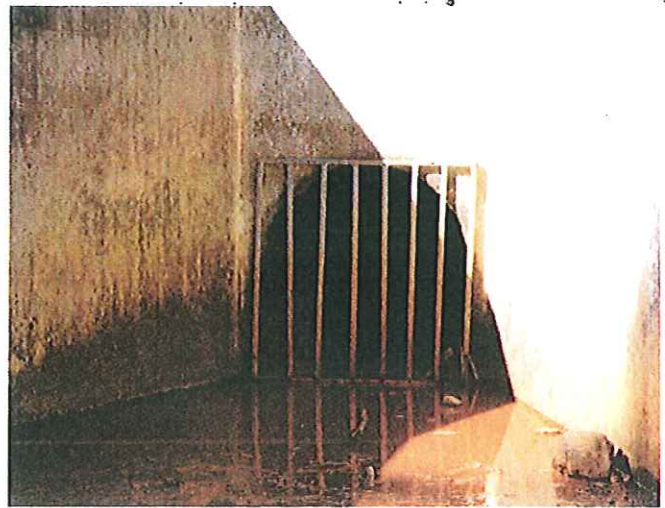
Photo No. 16: 42" CMP drain pipe outlet. Note small flow.
