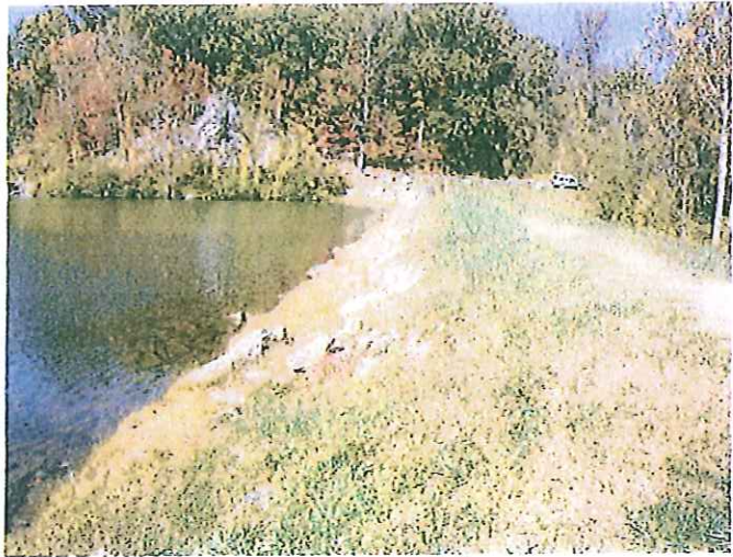
Photo No. 6: Upstream slope facing left.
