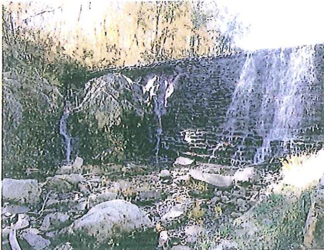
Photo No. 8: Principal spillway.
