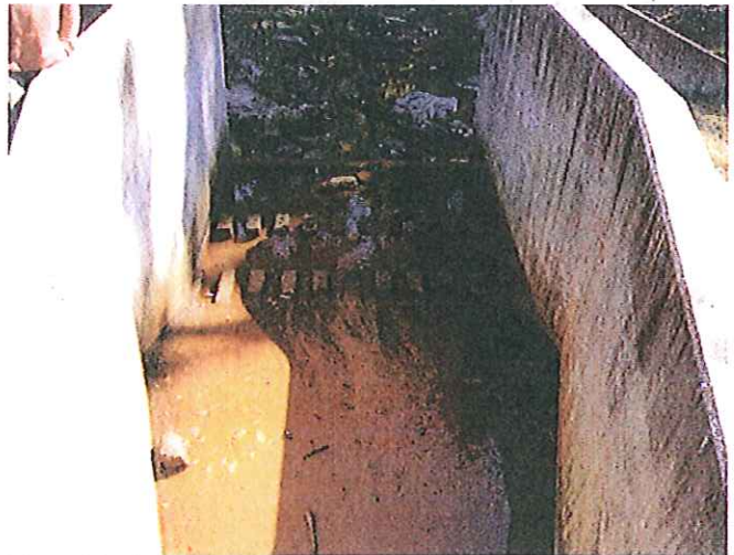
Photo No. 17: Principal spillway stilling basin and stream channel.
