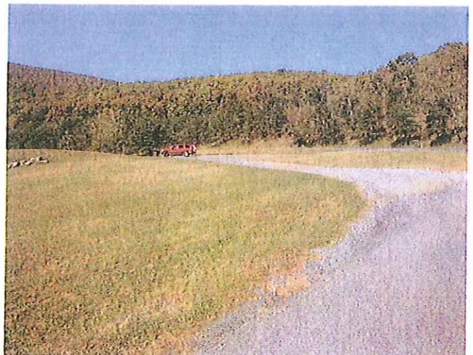
Photo No. 12: Emergency spillway facing upstream.
