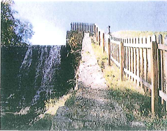
Photo No. 13: Left spillway guidewall facing upstream.
