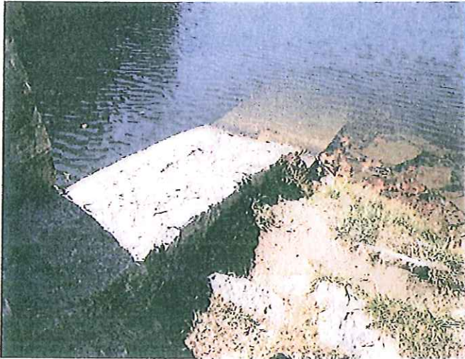
Photo No. 14: Left spillway guidewall.
