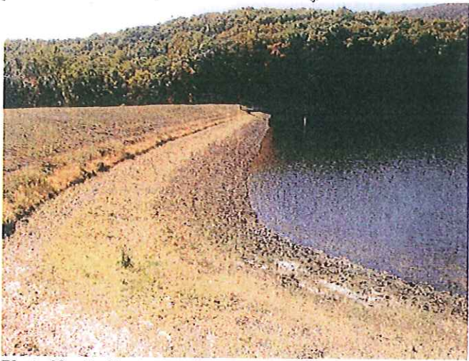
Photo No. 7: Upstream slope facing right.
