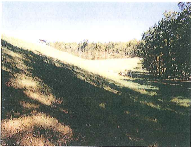
Photo No. 2: Downstream slope facing left.
