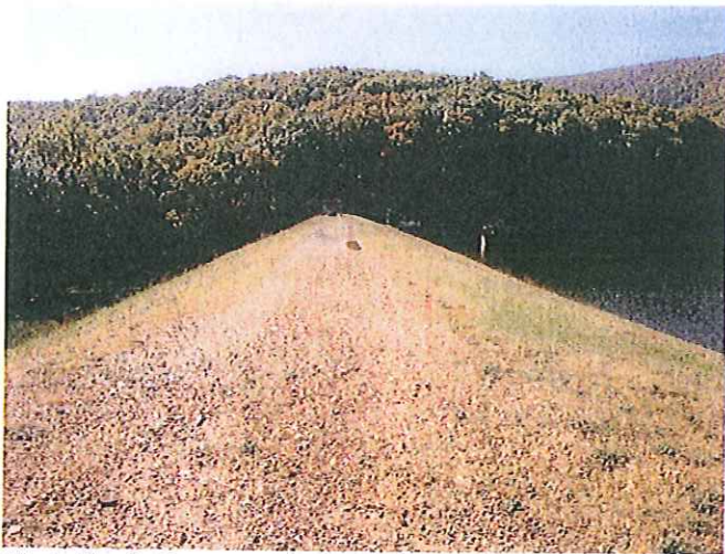
Photo No. 9: Dam crest facing right.
