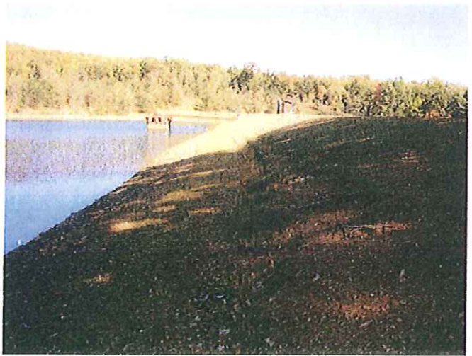
Photo No. 6: Upstream slope facing left.
