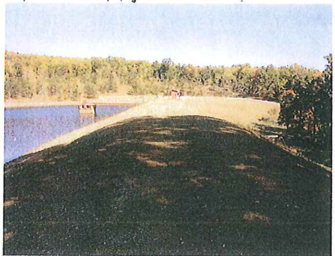
Photo No. 10: Dam crest facing left.
