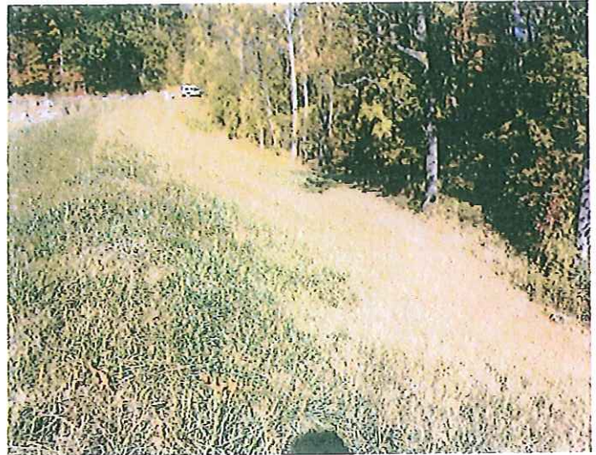
Photo No. 4: Downstream slope facing left.
