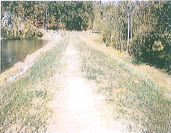
Photo No. 2: Dam crest facing left.
