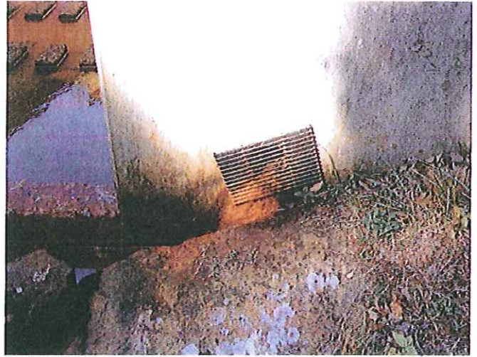
Photo No. 18: Left underdrain outlet.
