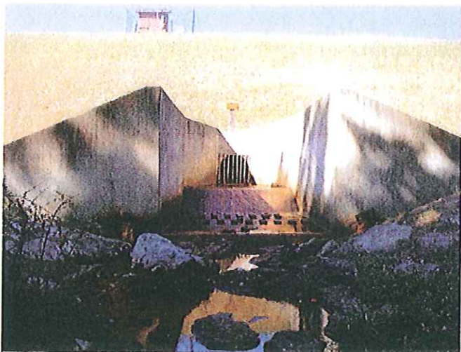
Photo No. 15: Principal spillway outlet structure.
