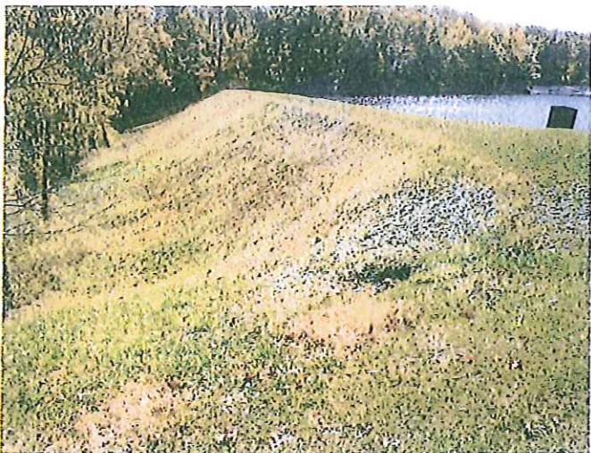
Photo No. 3: Downstream slope facing right.
