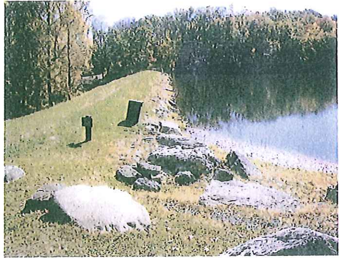
Photo No. 5: Upstream slope facing right.
