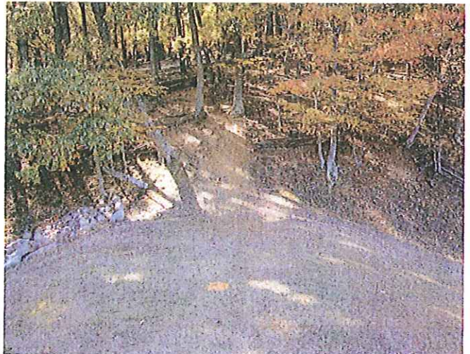
Photo No. 11: Erosion on slope to the right of crest.
