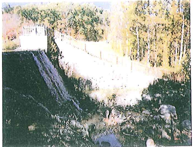
Photo No. 10: Left spillway wall.
