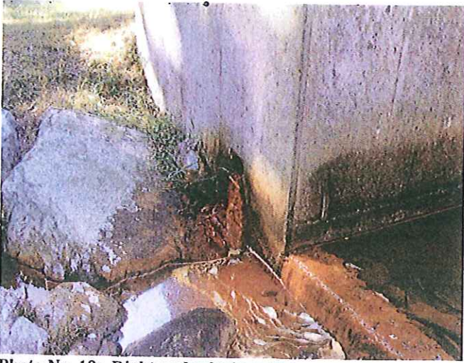
Photo No. 19: Right underdrain outlet.
