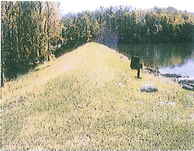
Photo No. 1: Dam crest facing right.
