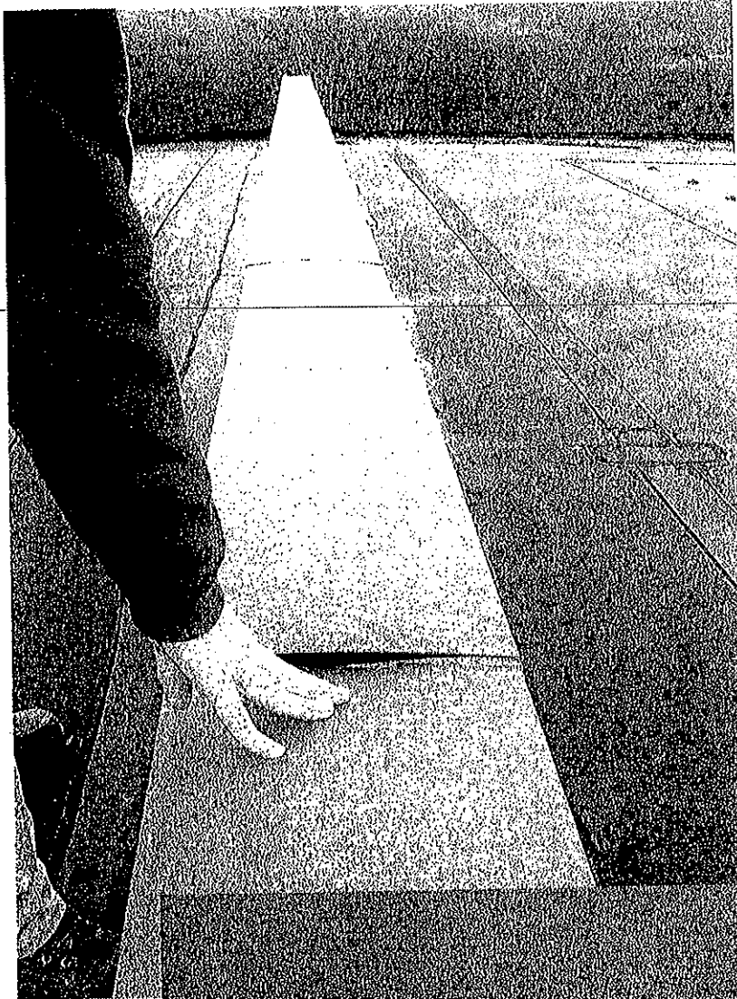
Photo 39. Open Joints in Cap Flashing Over Block Firewall on Raven Lodge
