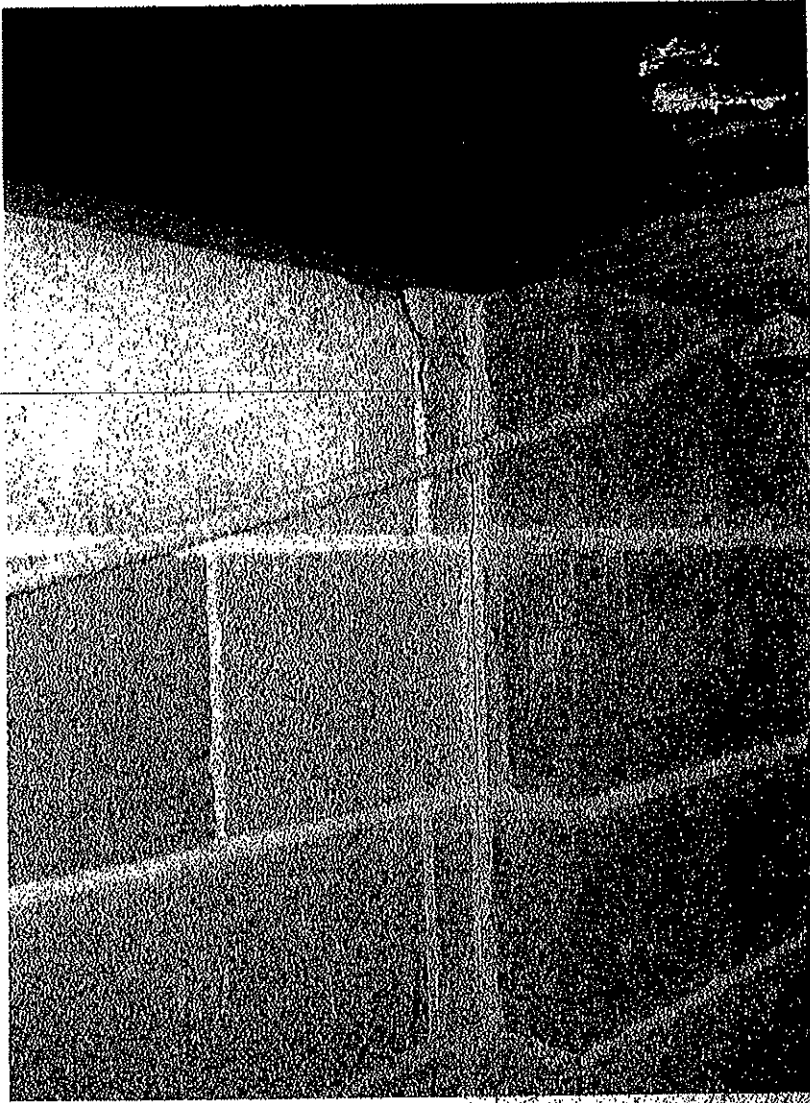
Photo 59. Another Pilaster Shows Evidence of Cracking at Exterior Foundation Wall
