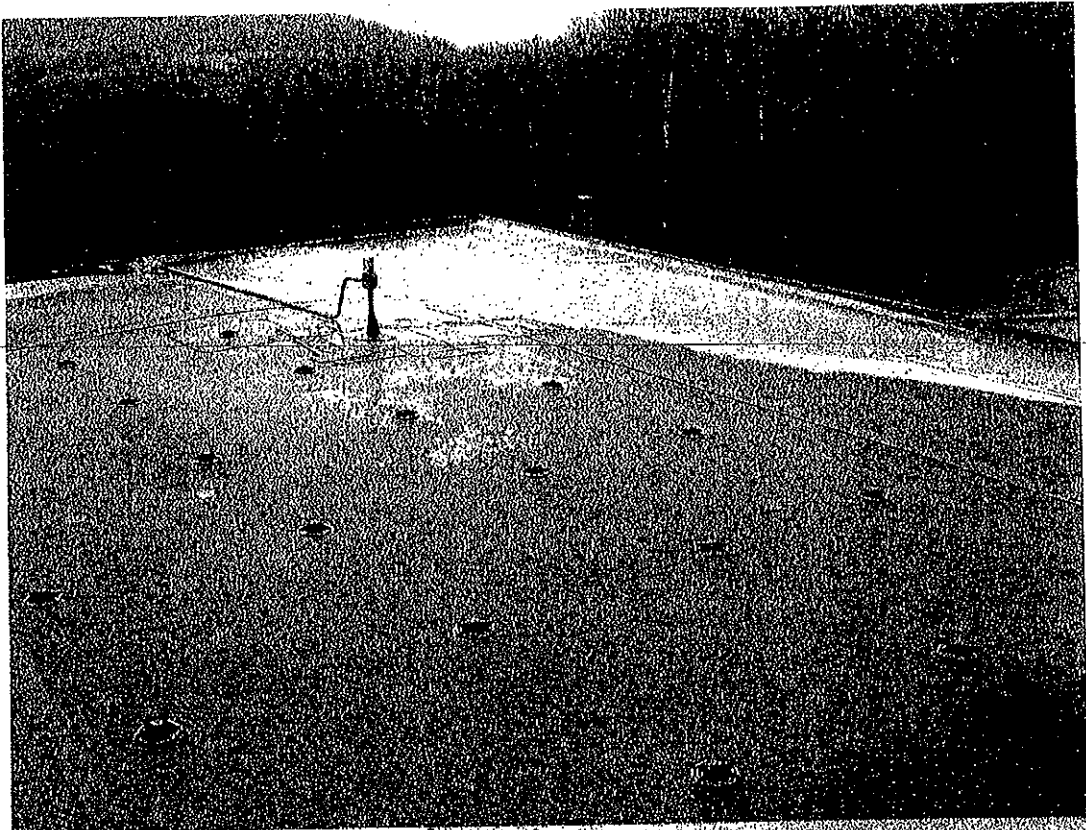
Photo 35. Water Ponding at Corner of Roof
