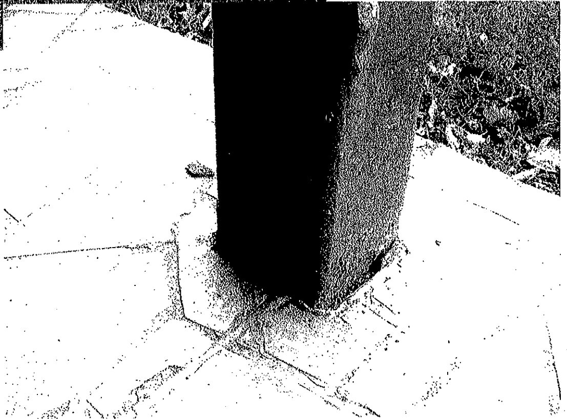
Photo 66. Deteriorated Steel Tube Column at Wild Goose Lodge
