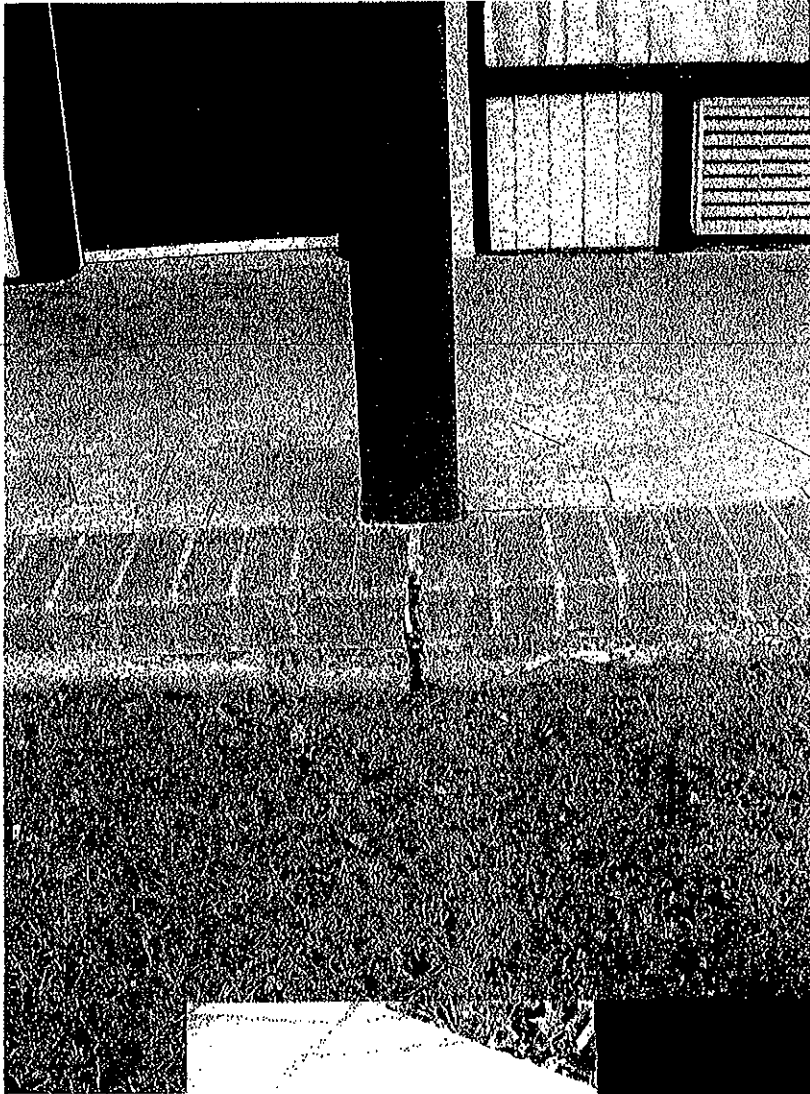
Photo 66. Deteriorated Steel Tube Column at Wild Goose Lodge
