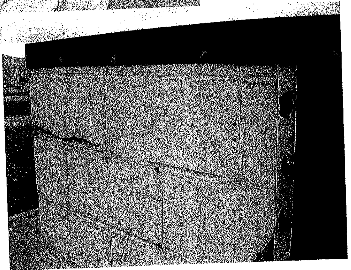
Photo 34. Mortar Joint and Block Cracking at Roof Level
