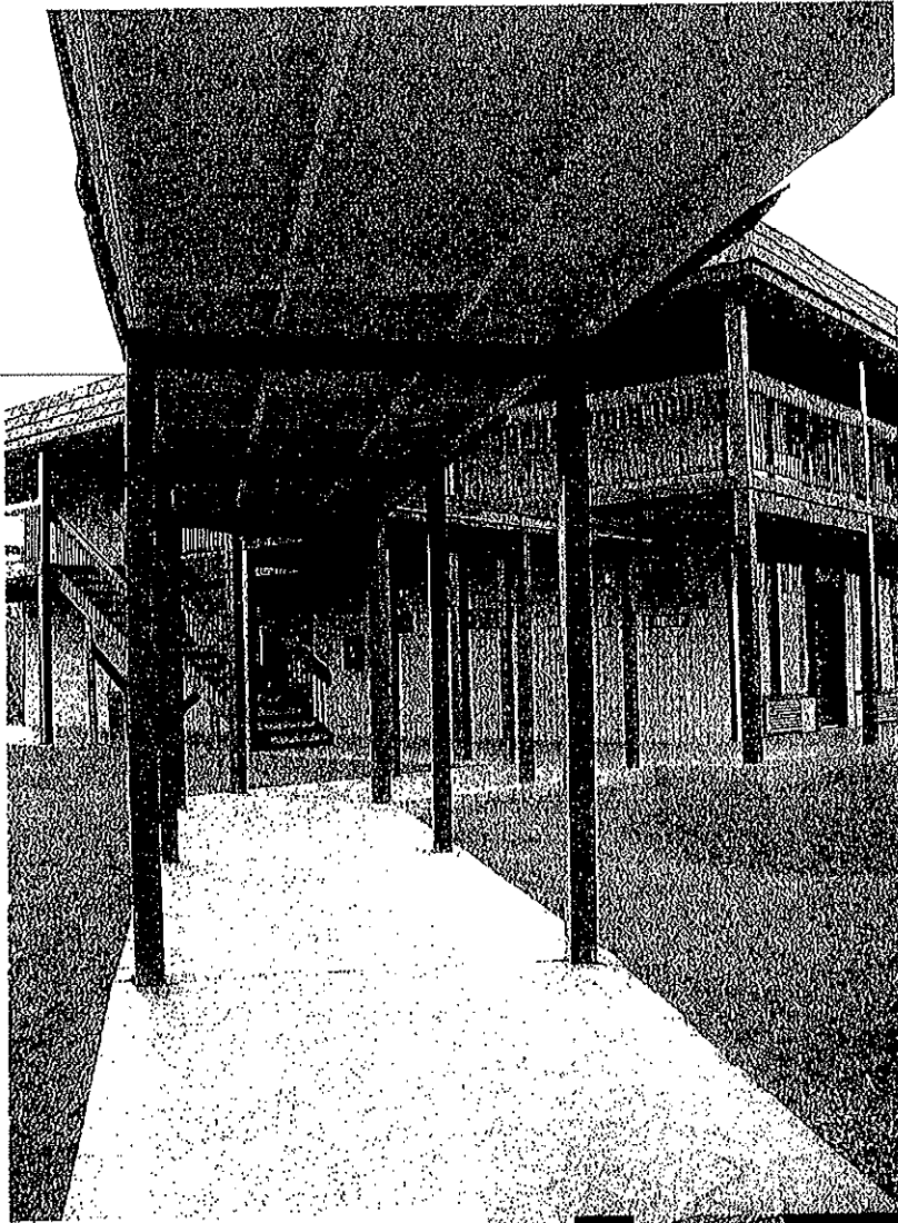
Photo 87. Another View of the Covered Walkway
