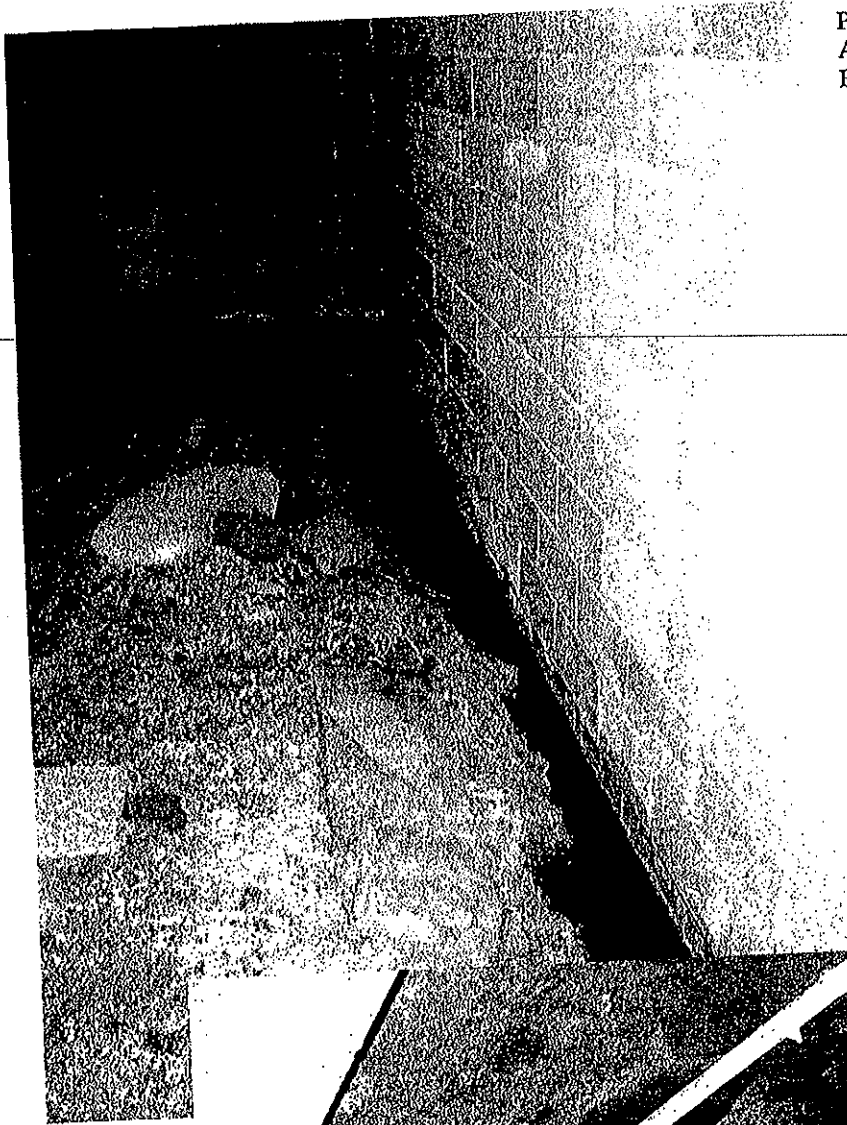
Photo 8. Mold on Vapor Bar- rier
