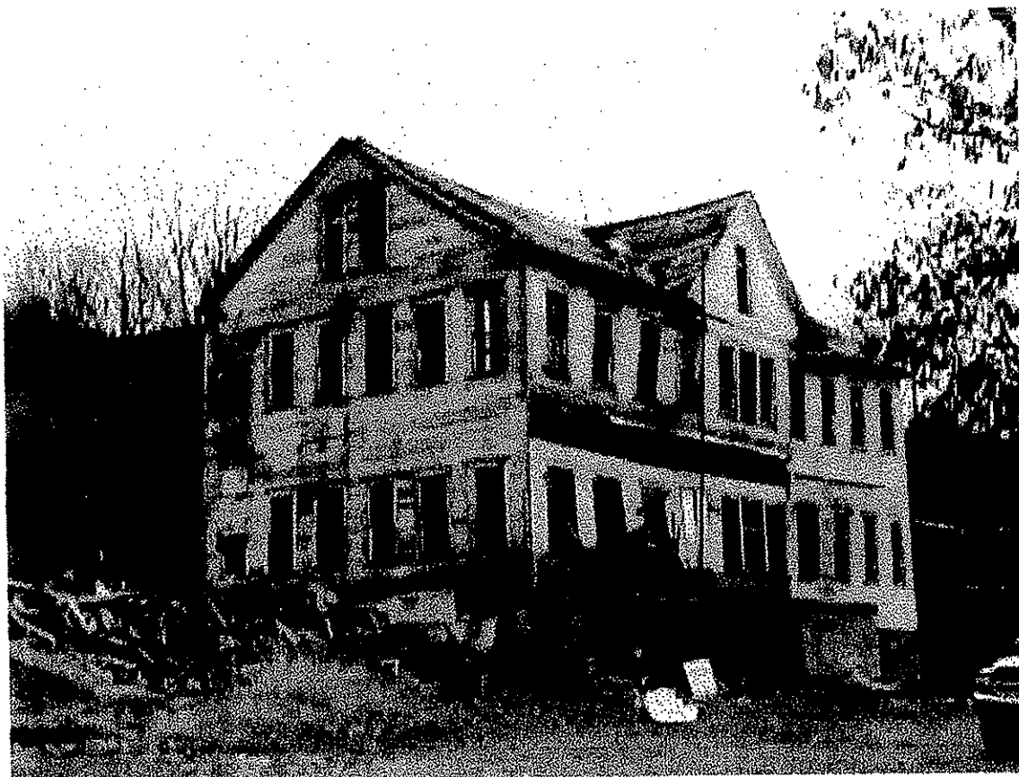
REMAINING SECTION MAIN BUILDING
