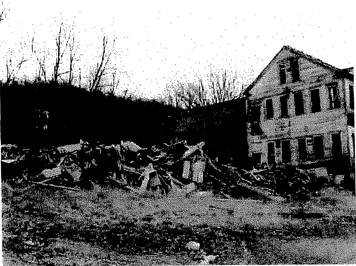
MAIN BLDG. SECTION AND ASSOCIATED DEBRIS PILE GYMNASIUM 3/17/08
