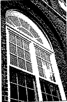
When the paint on the wood windows became too thick, it was removed and the window repainted. Photo: NPS files.
