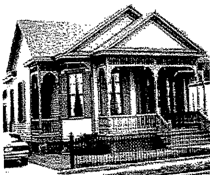
Decorative features were painted with a traditional oil-based paint as a part of the rehabilitation. Photo: NPS files.
