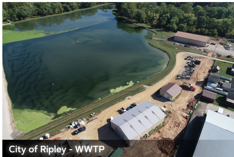
City of Ripley - WWTP
