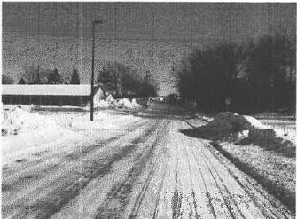
Burns through hardpack to break bond with road Breaking bond makes removal easier
