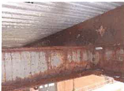
Evaluation of corroded structural steel framing elements
