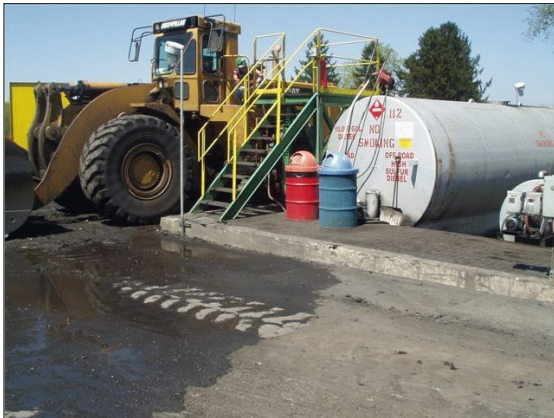
Aboveground Storage Tanks and Drums in Containment Area
