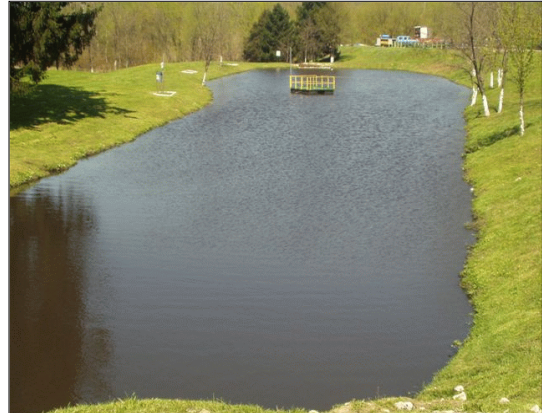
Settlement Pond Used to Control Storm Water Runoff
