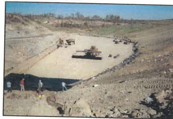
Construction of the 60-mil HDPE geomembrane over the prepared soil subgrade and excavation of perimeter anchor trenches.
