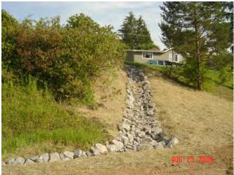
Erosion Repair – Rip Rap Armored Ditch
