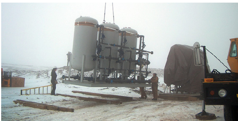
At the Gilt Edge Mine Site in South Dakota, CDM Smith conducted geochemical modeling to evaluate alternatives for addressing acid mine drainage. We designed, constructed, and operated a water treatment system that treated up to 160 million gallons annually.
