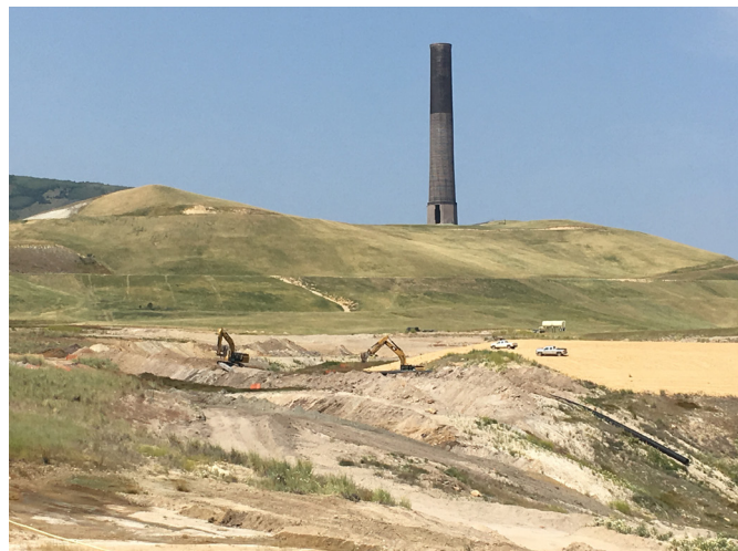
Borrow area development during closure of the Smelter Hill waste management area
