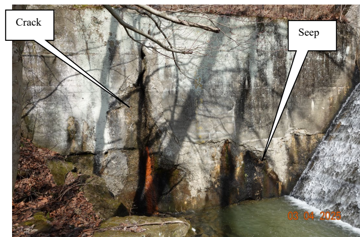
Face of right guide wall. Vertical crack, seep, and deterioration.
