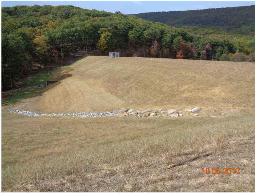
RESERVOIR DAM MODIFICATION, CACAPON STATE PARK (AFTER – NOTE BUTTRESS AT TOE TO CONTROL SEEPAGE AND IMPROVE STABILITY)
