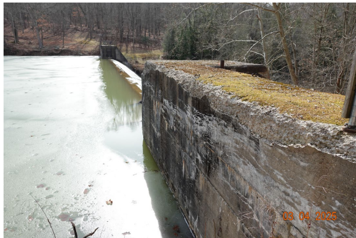
Right abutment. Note spalling.
