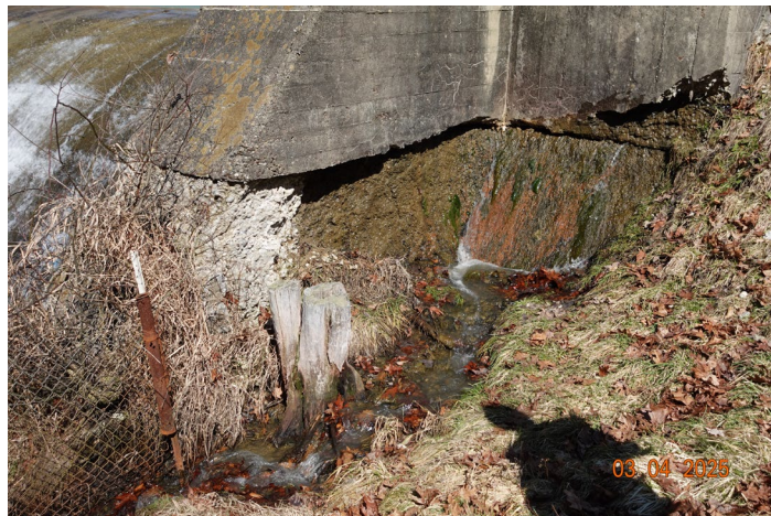
Gate well leak area and flow.
