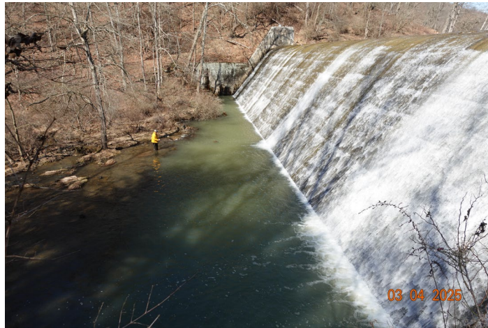
Spillway. Note lift lines. The lift lines exhibit minor spalling.
