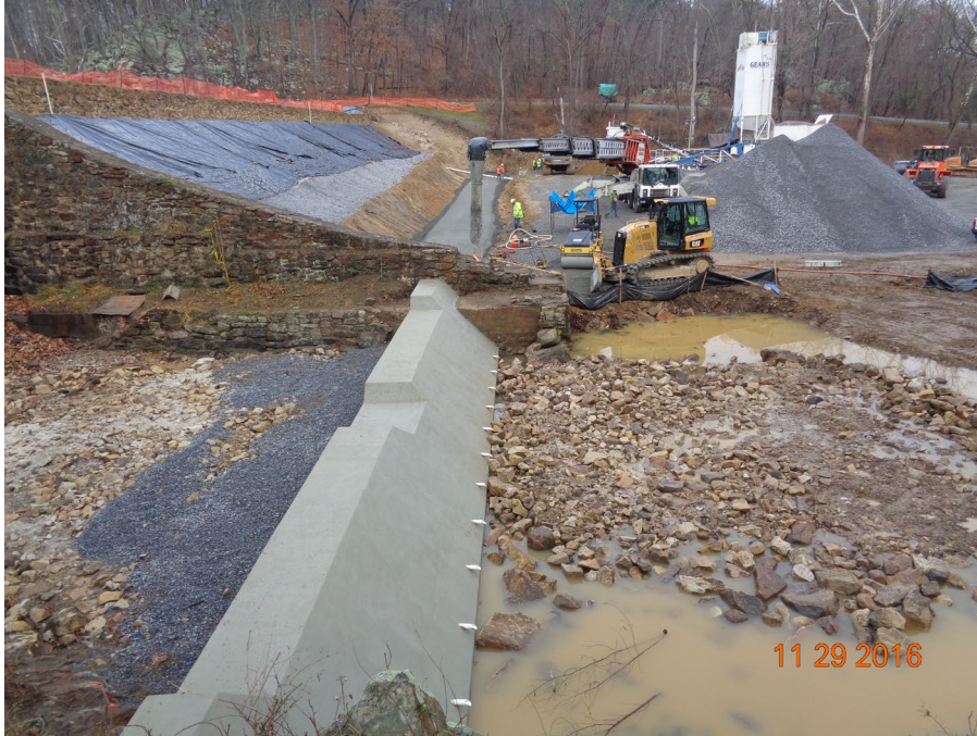
PARK DAM MODIFICATION (RCC PLACEMENT AND REINFORCED CONCRETE END DAM), CACAPON STATE PARK
