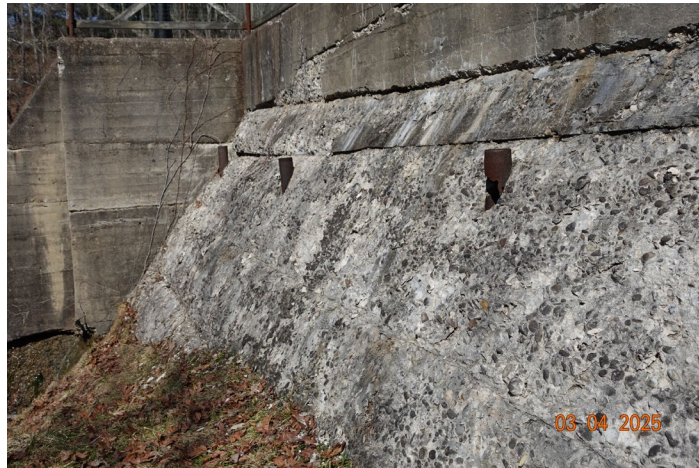
Left abutment spalling damage and joints.
