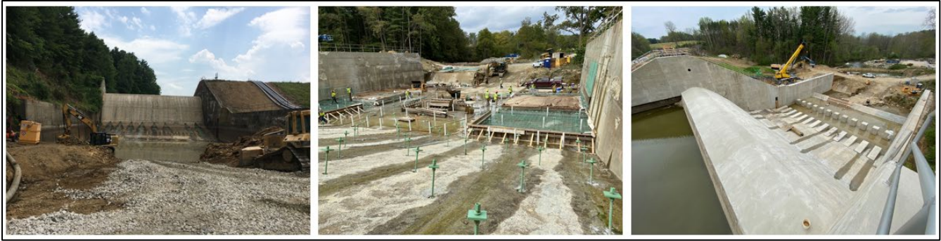
Photo of Concrete Overlay Project at Knox Lake Dam. Photo Before Construction (left), During Construction (middle) and After Construction (right).
