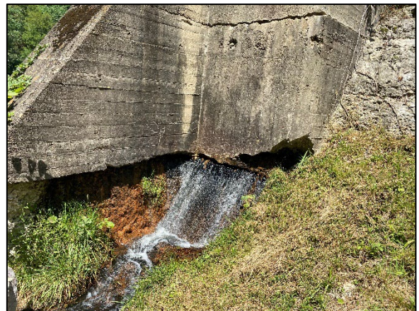
Figure 3: View of Spillway from Right Abutment (Left Photo) and Seepage at Left Spillway Wall (Right Photo)
