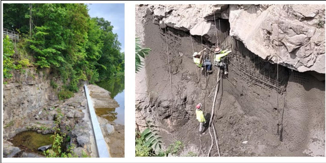
Photo of Rock Spillway Improvements at Cobun Creek No. 1 in Monongalia County, WV. New Overflow Weir (left) and Guniting Rock Protection (right).
