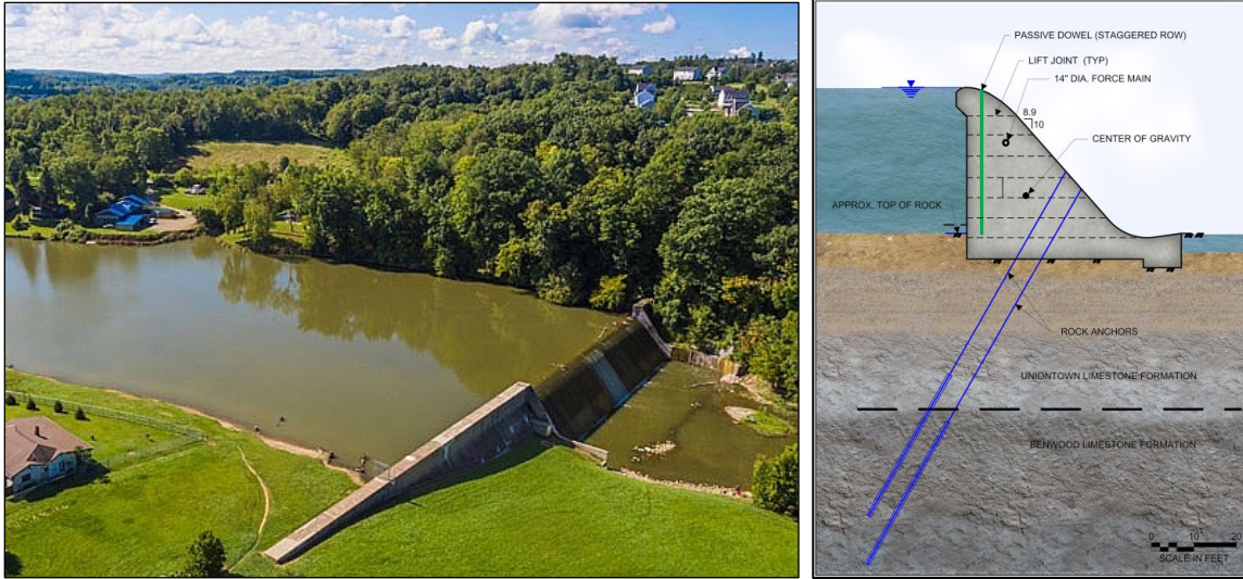
Photo of Canonsburg Dam After Stability Improvements and Select Concrete Repairs (left) and a Figure of the Rock Anchors Installed in the Concrete Gravity Dam (right)
