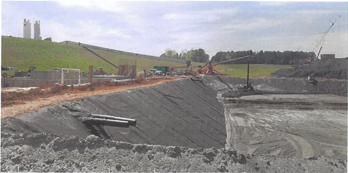
Pugmill mixing plant (top left) mixing RCC, RCC conveyance and placement over a sand cushion layer protecting the in-place dual membrane liner with geotextile fabric and filter fabric. Two of this project's 20 reinforced concrete structures can be seen to the left of the basin.
