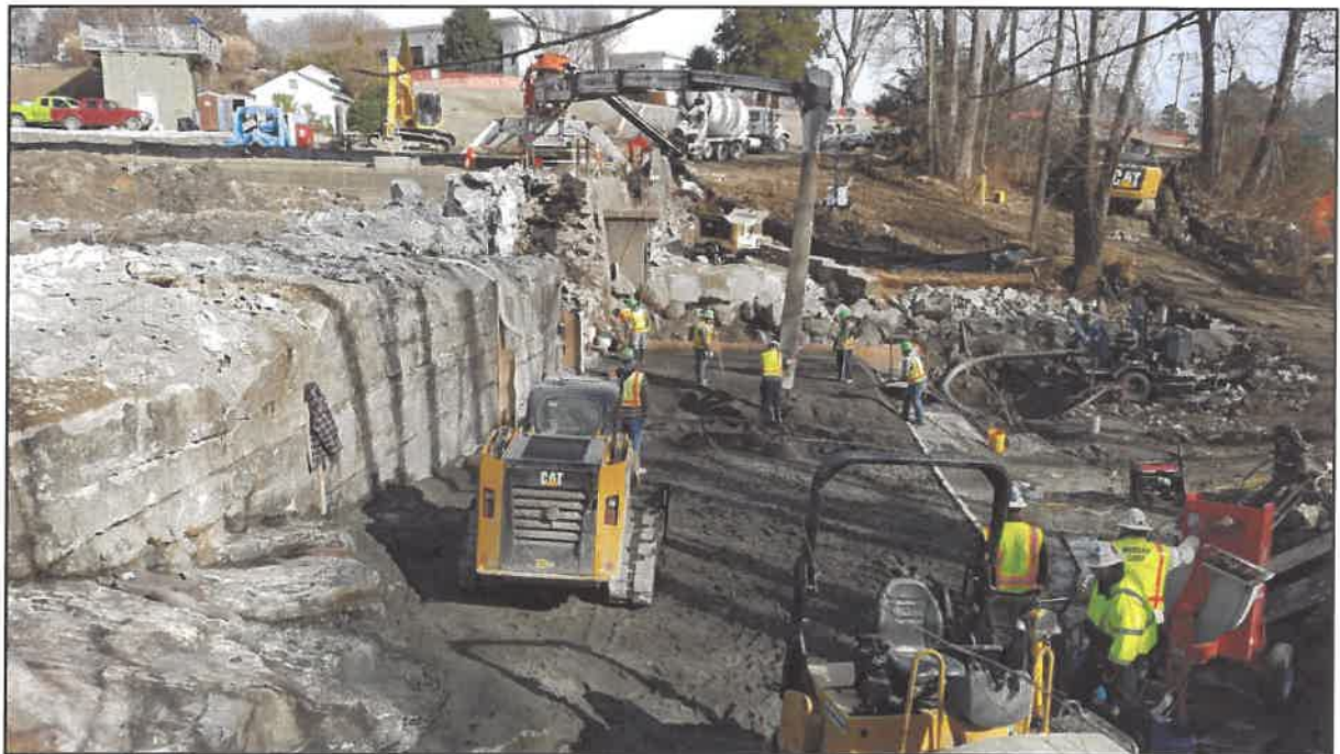
RCC conveyance and placement
