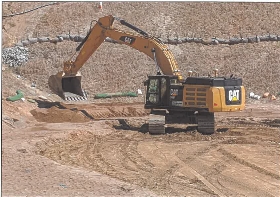
Filter drain construction at Lookout Shoals Dam Project
