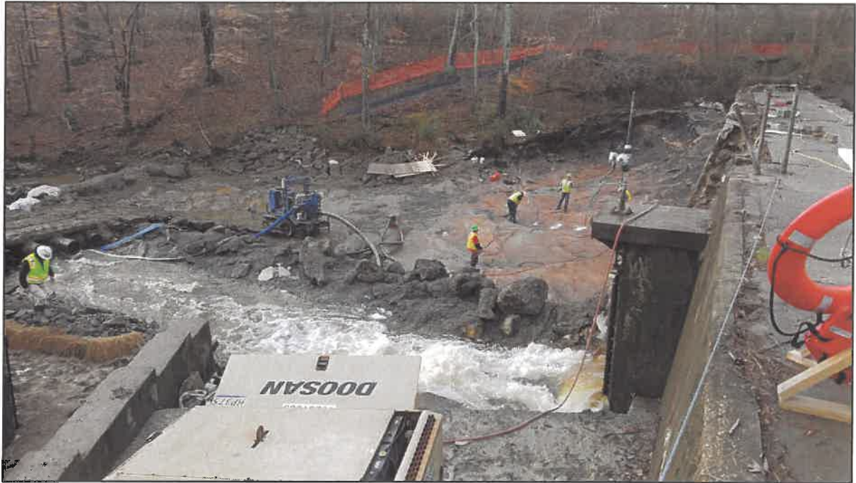
Water diversion using existing culvert and a flume while preparing the foundation bedrock to build the right abutment section of the new dam
