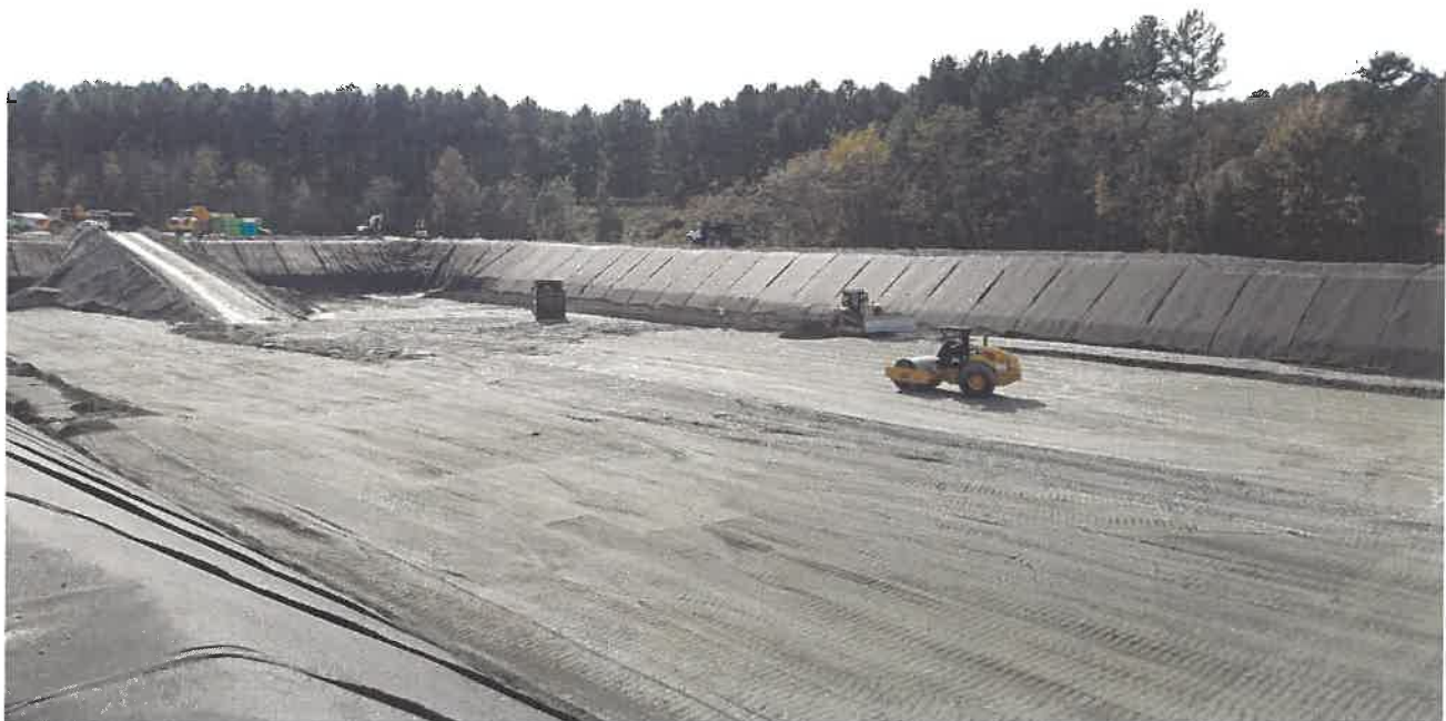
RCC spreading and compaction at Plant Mayo Water Redirect Holding Basin
