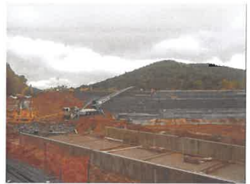
Final stages of RCC placement before grassing and topsoil.
