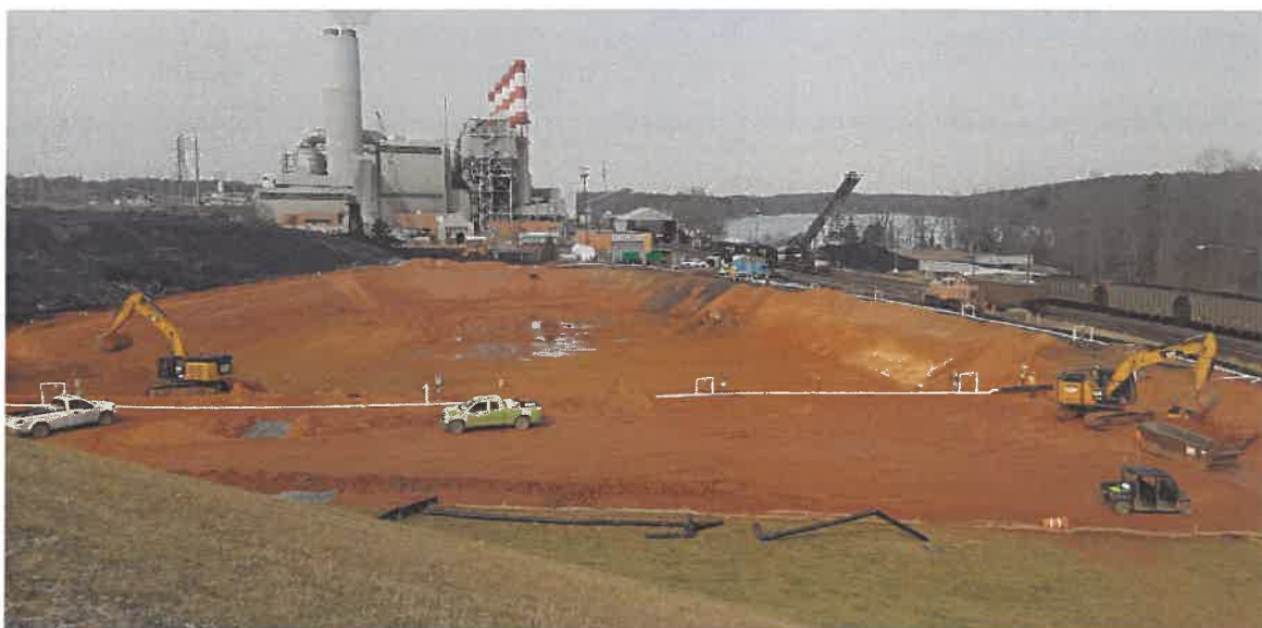
Excavation for holding basin with perimeter dewatering pumping system in place to lower the water table during construction at Plant Allen Steam Station
