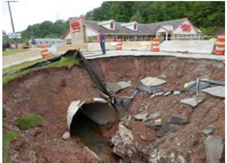
During a storm event in December 2015, a section of 120 inch pipe collapsed in the parking lot of the Golden Corral in Cross Lanes WV. TERRADON was retained by the restaurant owner, Platinum Corral, to determine the best method of repairing the pipe while ensuring the safety of the restaurants customers.
