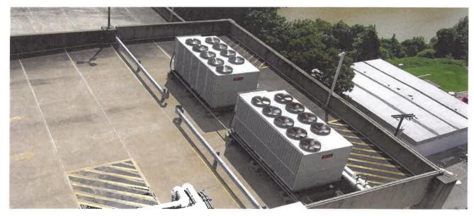
**Charleston Coliseum & Convention Center (2015)** – Replace entire MEP infrastructure three 1,000 ton chillers and cooling towers, three 8,000 mbh gas condensing boilers, approximately ten VAV AHU's, approximately 10 large single zone VAV AHU's.
