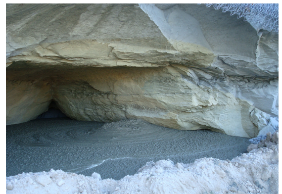
Example of RESPEC remotely constructing a barrier with zero slump grout and then backfilling with high slump grout.
