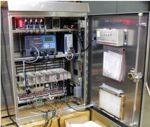
NEMA TS2 Type 2 12 Position Cabinet Assembly
