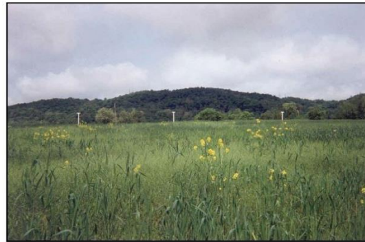
Post construction photograph showing revegetated landfill cap.
