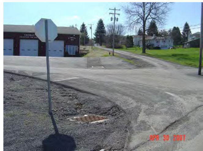
New Storm Drains and Catch Basins
