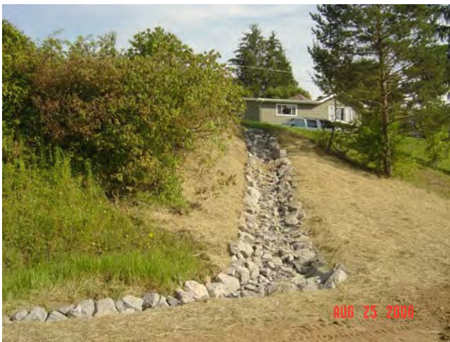
Erosion Repair – Rip Rap Armored Ditch
