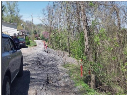
Slide Before Repair
