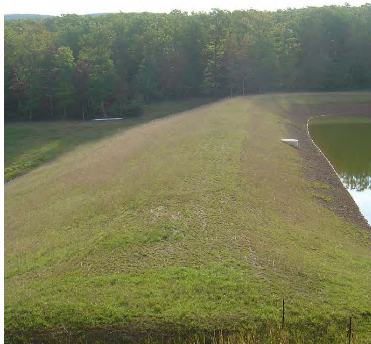
WILSON DAM MODIFICATION, HAMPSHIRE CO., WV
