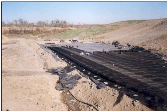
HDPE drainage net was installed as the leak detection layer above the 60-mil HDPE geomembrane.
