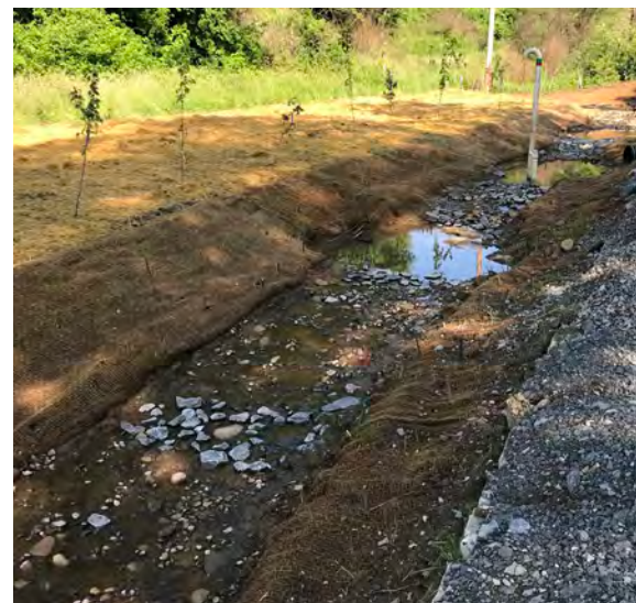
Impacted Stream Post Construction
