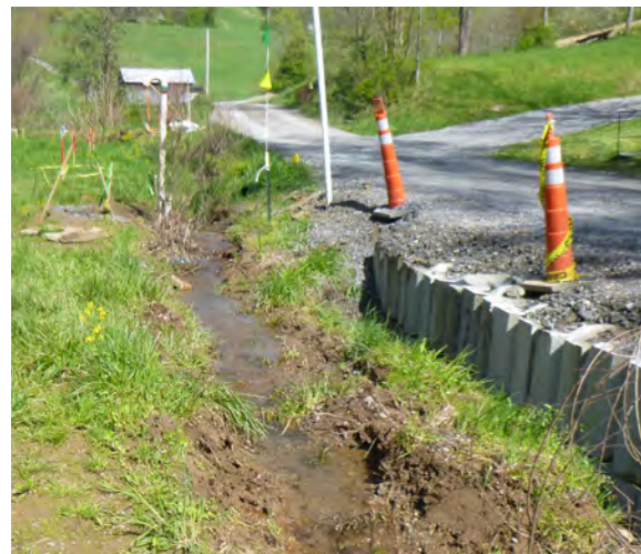
Impacted Stream Before Construction
