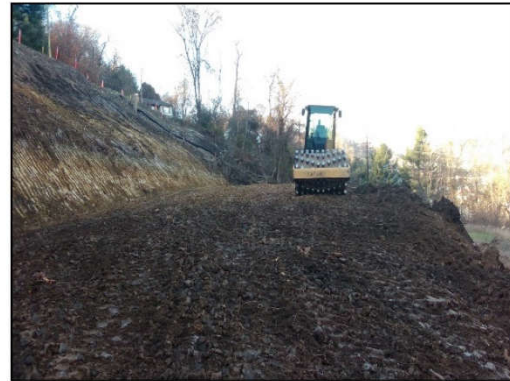
During Construction of Repair
