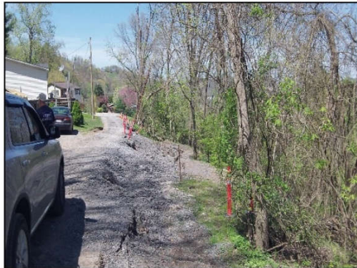
Slide Before Repair
