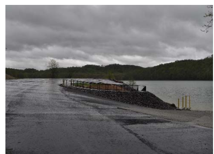
Tygart Lake State Park Parking Lot Expansion
