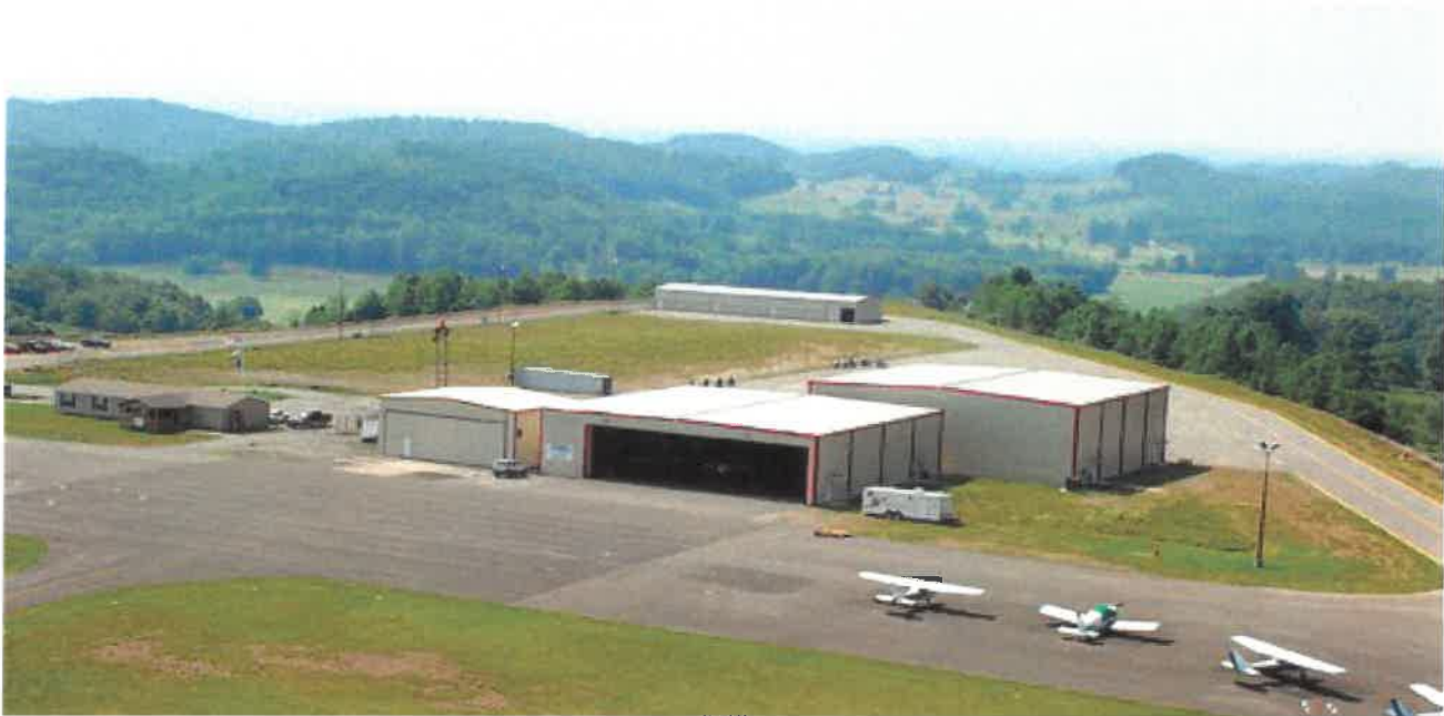
Buckhannon Upshur Airport Authority New Airport Hangars 40 West Main Street Buckhannon, West Virginia 26201
