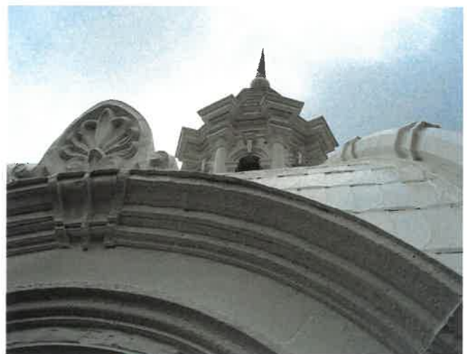
Dome Restoration Detail
