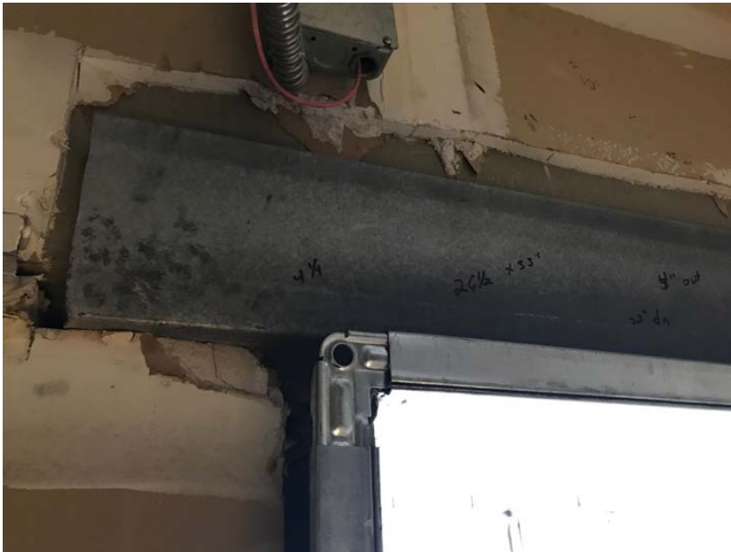
Interior view of the lintel above duct penetration at 3 rd floor.
