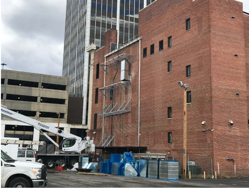
Back of the building with new steel supports and ductwork installation has started.
