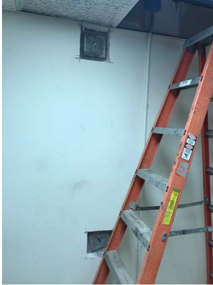
3 rd floor with exterior steel frame thru-bolts visible.
