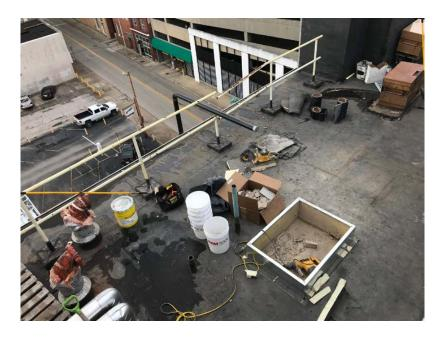
Contractor is making penetration thru the roof for ductwork.
