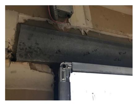
Interior view of the lintel above duct penetration at 3<sup>rd</sup> floor.
