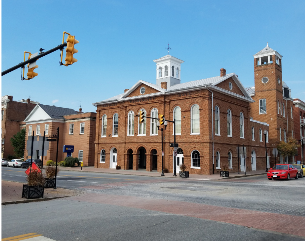
July 2016 - Near completion of Historic Rehabilitation - note complete facade reconstruction.
