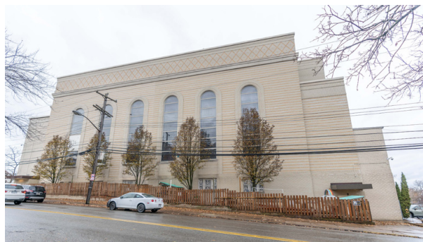
Beth Shalom Façade and Building Envelope Study
