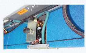
4 Ton externally equalized, thermostatic expansion valves that precisely control refrigerant and prevent liquid slugging to the compressor(s) or starved evaporator(s)
