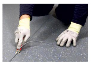
For finishes, move aside the trimming guide. Don't forget to regularly change the blade.
