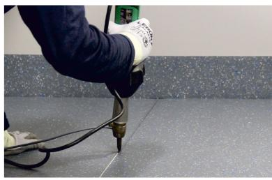
For corner weld, use a CA72 welding rod.
