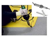
Hot weld the logo to the main flooring material using CR50. Recommended tools: Welding Gun Leister Triac'S (E8090002), Anti-Glaze Rapid Nozzle 4-5mm (E8100002)
