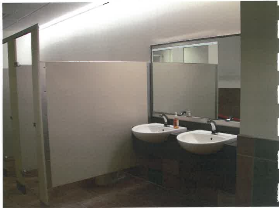
WVSP Detachment renovation
