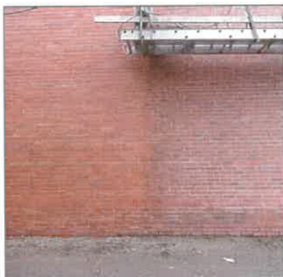
Photo Showcasing Masonry Restoration
