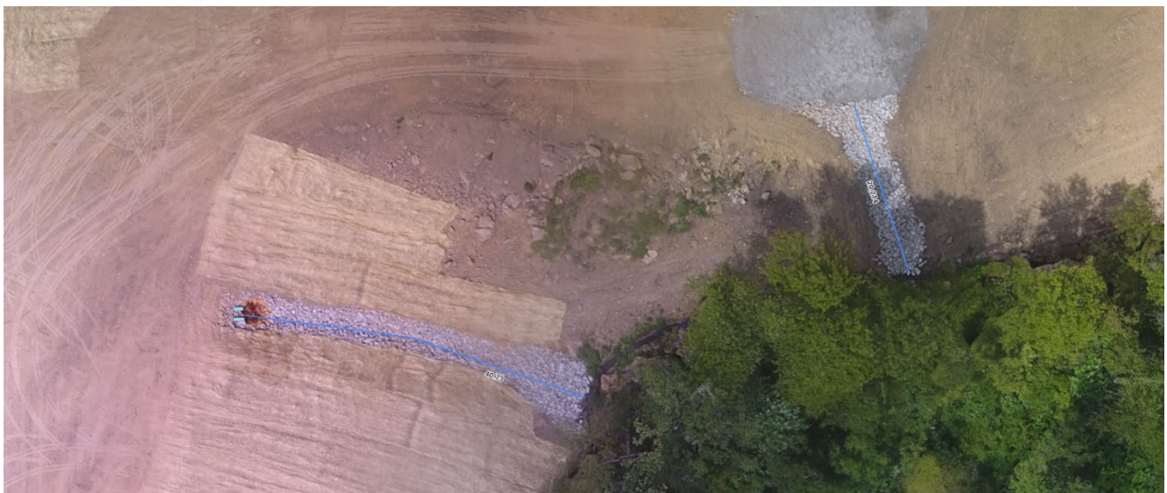
Canyon Run AML – As-Built Monitoring
