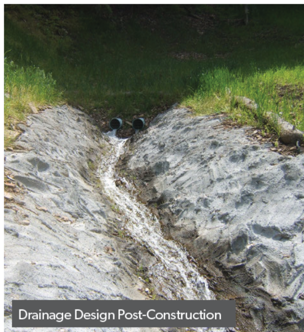
Drainage Discharging into a Stormwater System
