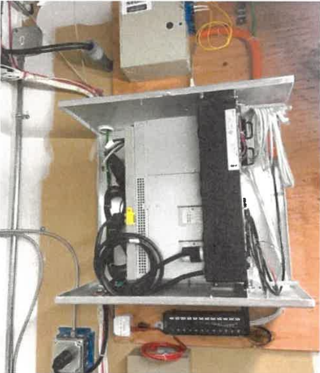
Completed installed cabinet (door open)
