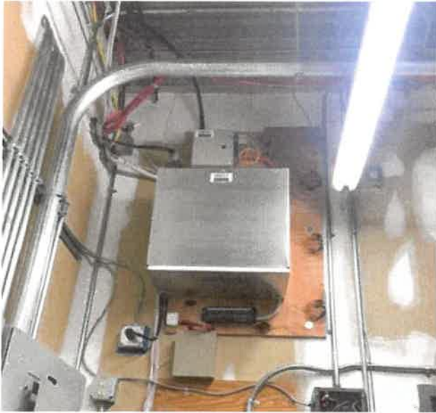
Completed installed cabinet (door closed)
