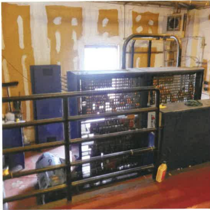
Machine Room Before Modernization
