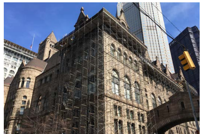
Construction under way, summer 2018—Scaffolding to the eave of the roof line; each week a crane is brought in to unload demo'd materials and load new tile to the top platform.
