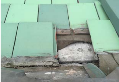
Ludowici tile fabricated to match original signature color; roof restoration in progress
