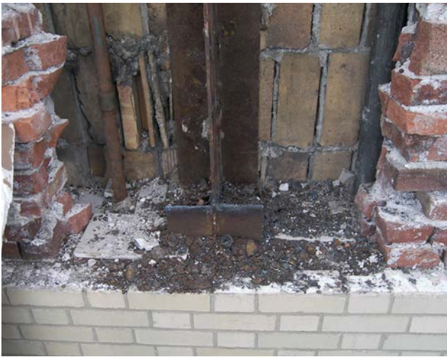
Forensic field investigations revealed significant deterioration of masonry and steel at the terra cotta frieze, balustrade, and lintels above the windows.
