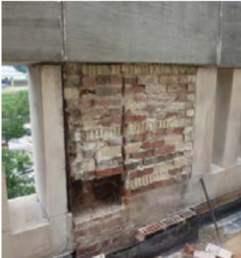
Parapet during exploratory demolition
