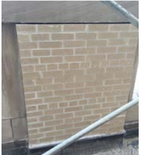
Reconstructed parapet mitigates water infiltration
