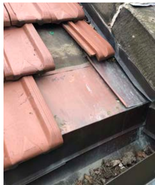
SGH and PWWG team members removed roof tiles to investigate existing conditions while the building was fully occupied.
