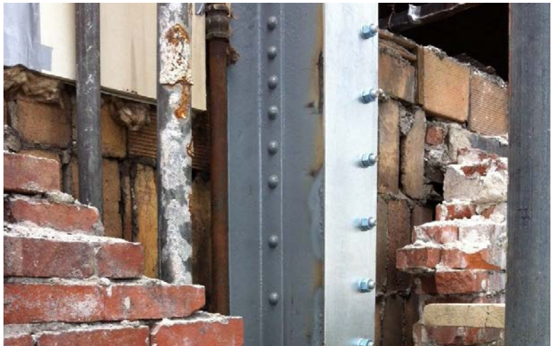
Forensic field investigations revealed significant deterioration of masonry and steel at the terra cotta frieze, balustrade, and lintels above the windows.
