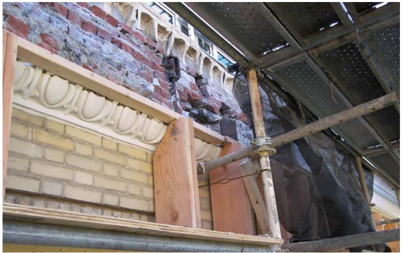
Forensic field investigations revealed significant deterioration of masonry and steel at the terra cotta frieze, balustrade, and lintels above the windows.
