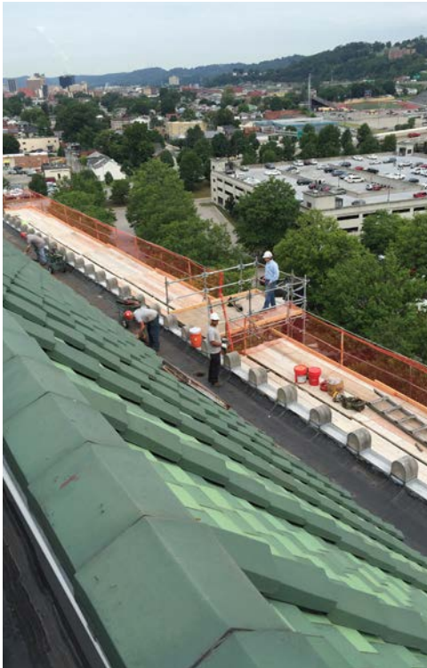
Ludowici tile fabricated to match original signature color; roof restoration in progress
