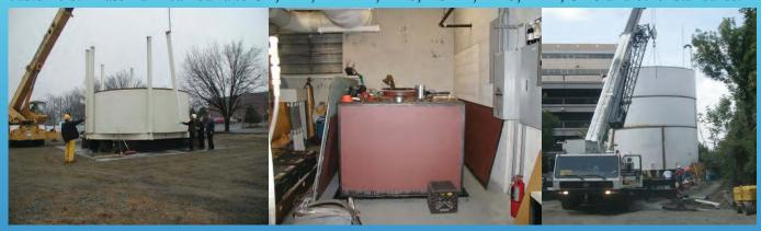
*Chilled Water Tanks* - Chilled Water TES (Thermal Energy Storage) tanks have been used in data centers and technology companies to bring about a cost effective answer to power outages utilizing back-up resources. Mass Tank has successfully utilized their own patent pending designs to build tanks that are either shop built or field fabricated.
