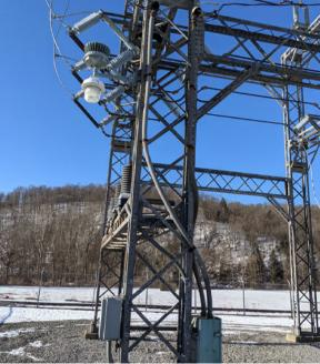
GAI designed for an Automatic Transfer Switch (ATS) replacement at a substation for a confidential client. The existing outdoor ATS had failed and the client requested a replacement along with additional alarming. GAI performed a site visit and designed for the mounting, placement, wiring schematic and SCADA alarms per client request in accordance with their standards. GAI also assisted with construction support and provided engineering guidance during installation.
