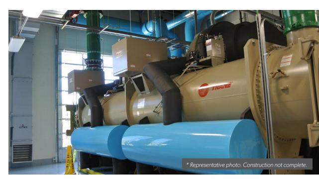
The project scope of services involved designing a new 25,000 ton chilled water plant for a district energy company in Florida. GAI's scope included site layout, design of the building, sizing of all equipment, writing all specifications, and all structural, mechanical and electrical engineering.
