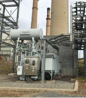
GAI designed for an Automatic Transfer Switch (ATS) replacement at a substation for a confidential client. The existing outdoor ATS had failed and the client requested a replacement along with additional alarming. GAI performed a site visit and designed for the mounting, placement, wiring schematic and SCADA alarms per client request in accordance with their standards. GAI also assisted with construction support and provided engineering guidance during installation.
