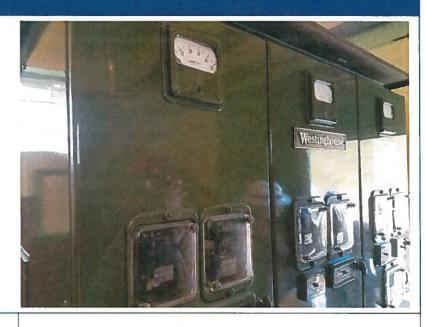
Miller Engineering worked with Potesta and Associates to design upgrades to the automation of the seventeen floodwall pump stations which serve the city of Huntington, WV. These stations consist of both storm water and sewage pumps. The pump stations will utilize SCADA units with cellular capability to monitor and
