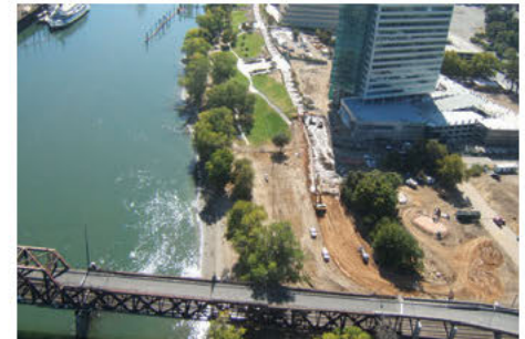
Natomas Levee – slurry wall installation
